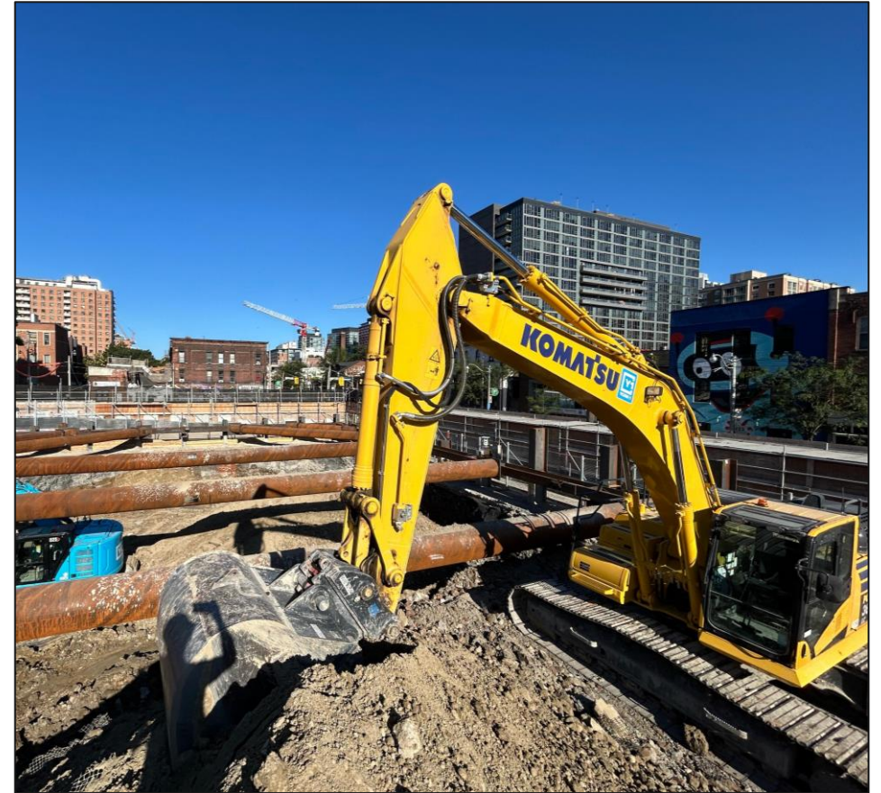
Excavation and spoils removal in the east (station building)
