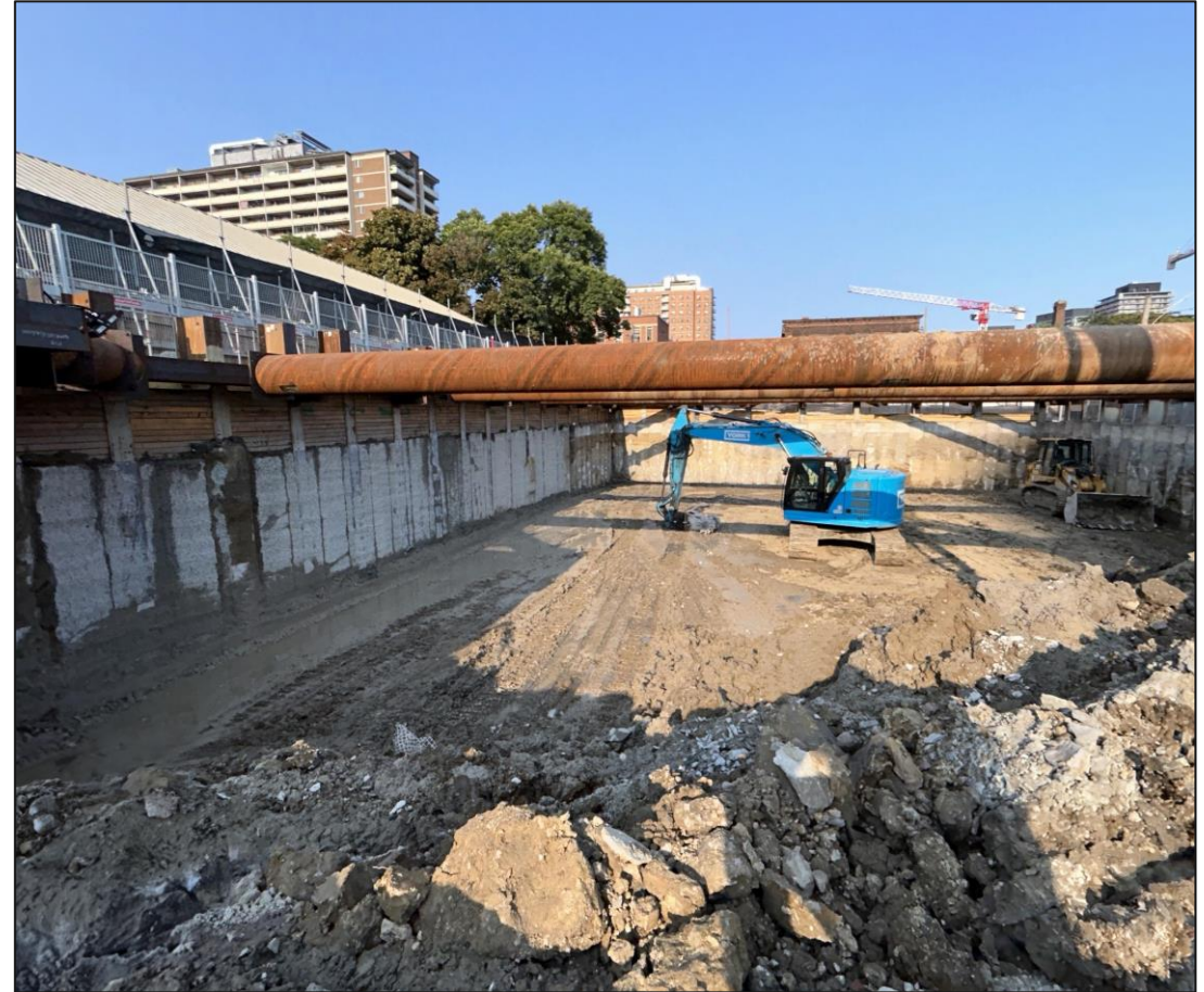
Excavation and spoils removal in the east (station building)
