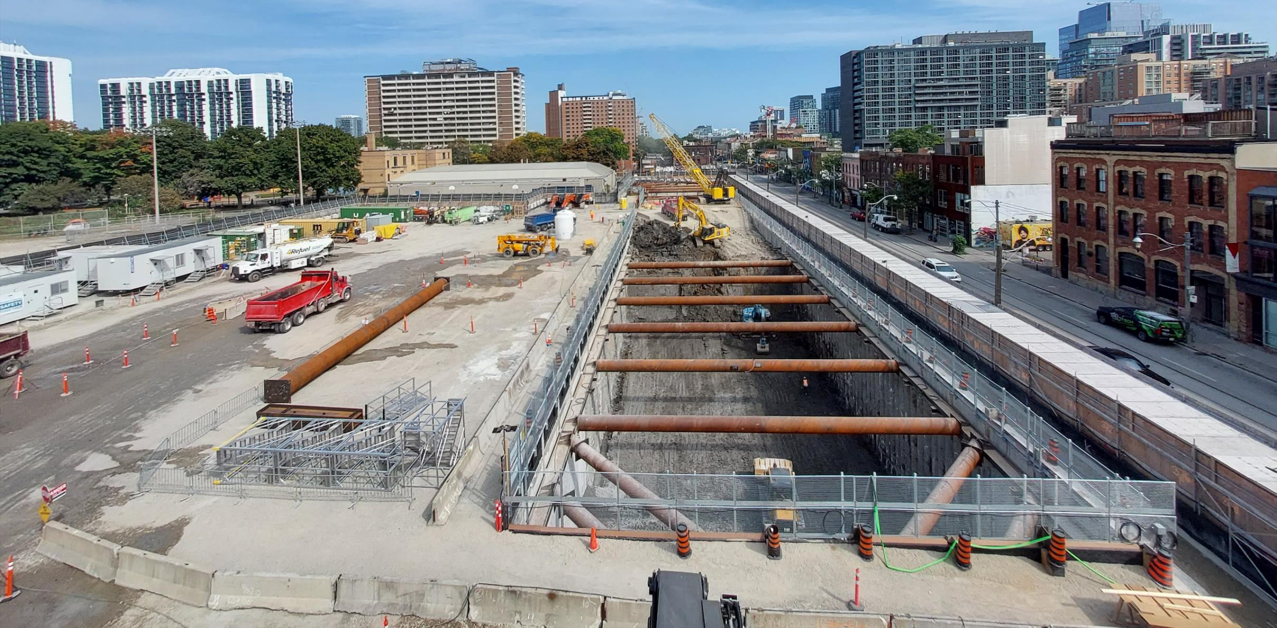
Struts and walers installation in the west (roof slab)
