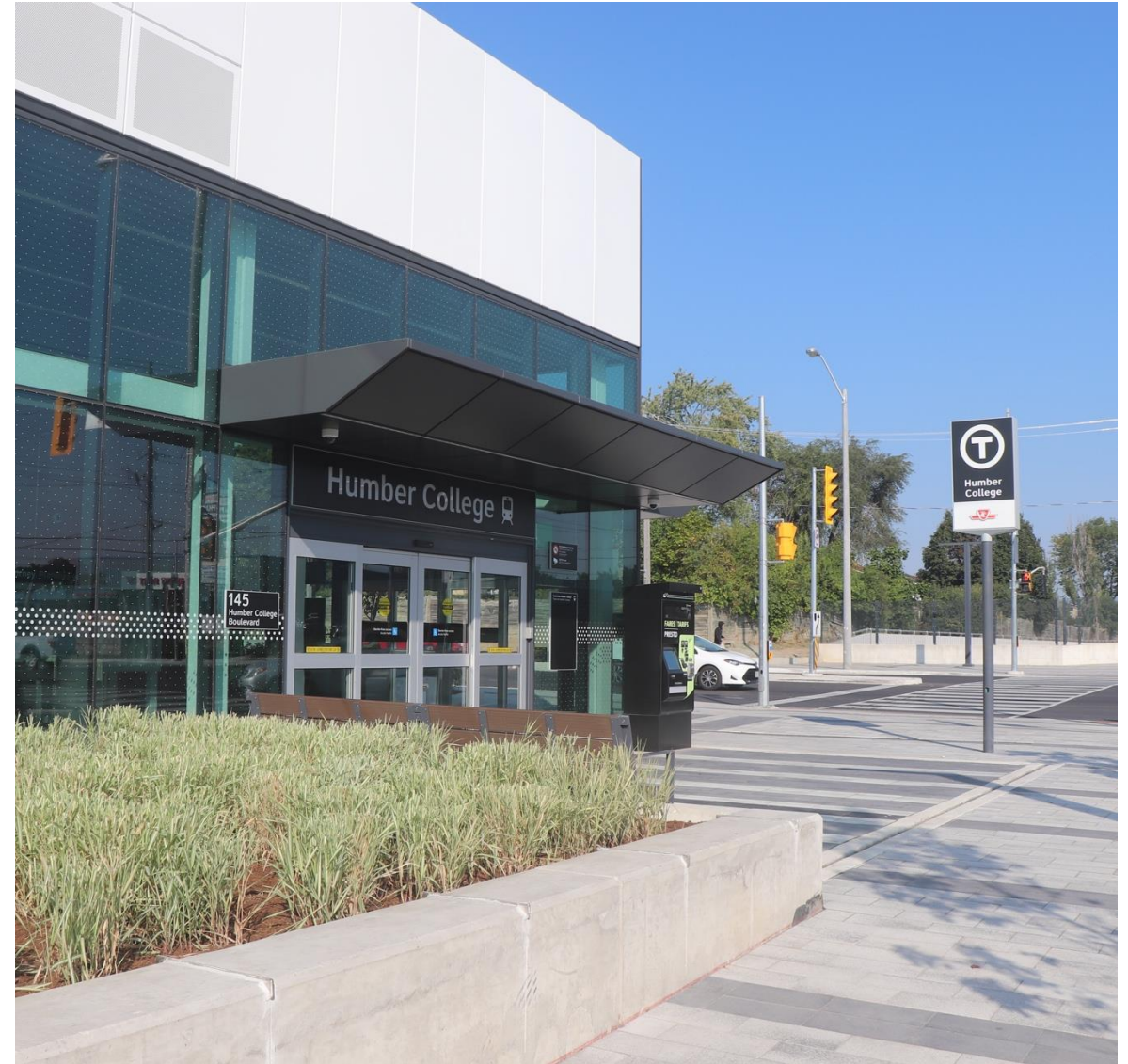
Photo: Humber College station exterior north building, east entrance. 2024.09.20
