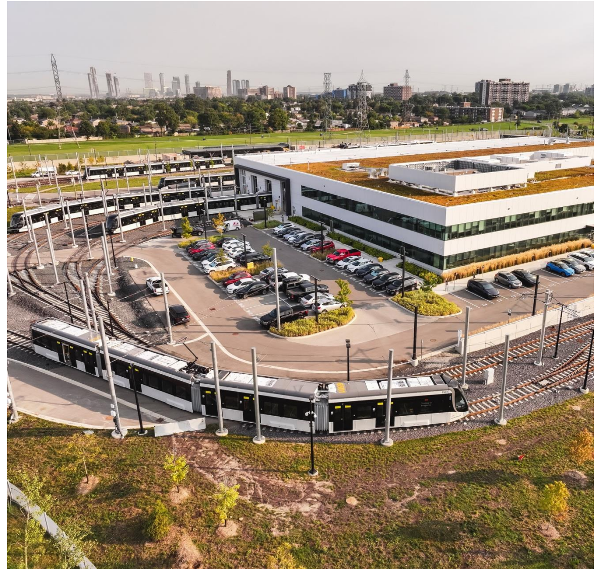
Photo: Maintenance and Storage Facility, northeast aerial view. 2024.09.12
