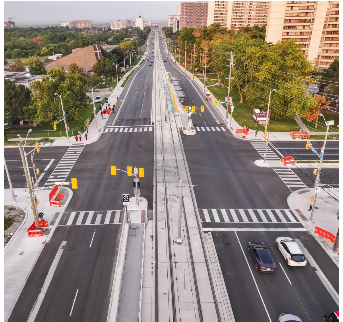
Photo: Finch Avenue West and Sentinel Road, aerial view west 2024.09.12
