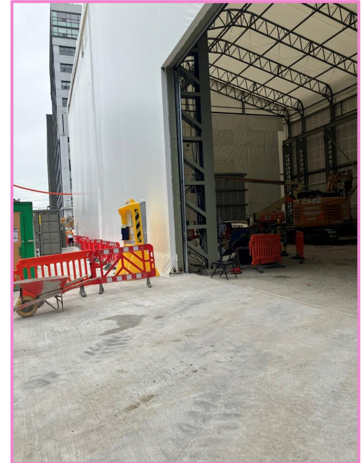
Paved worksite & acoustic shelter to reduce dust.& noise
