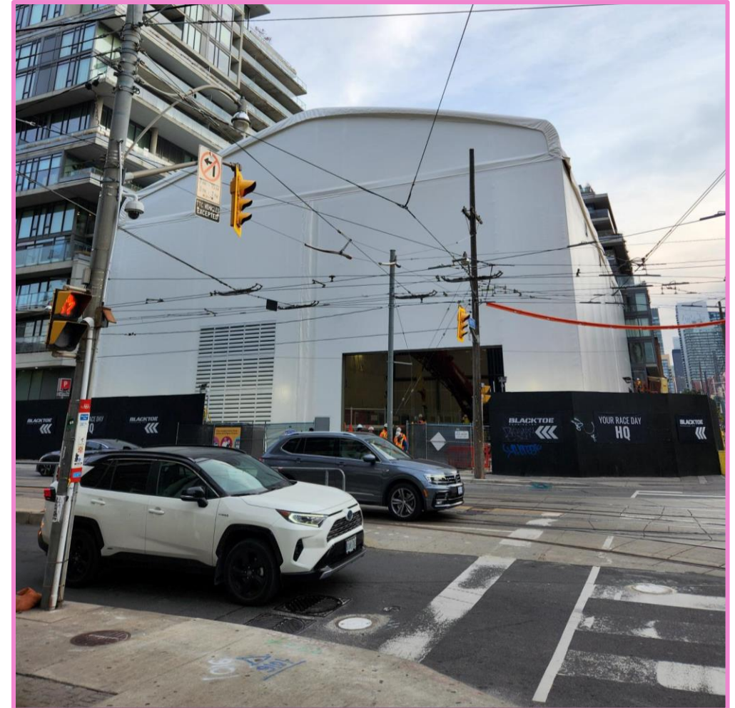
Exterior of the acoustic shelter, looking east from the NW corner.
