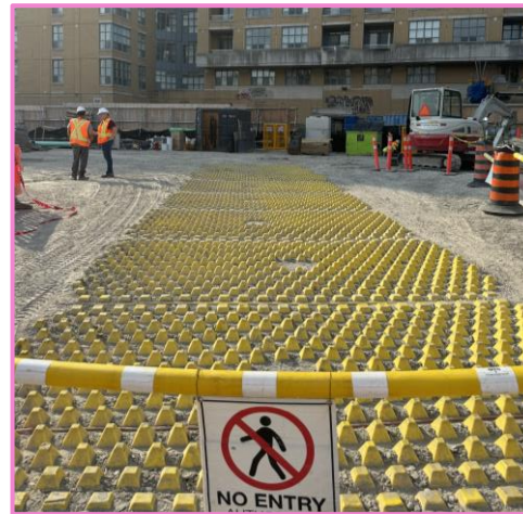
Example of mud mat installed
