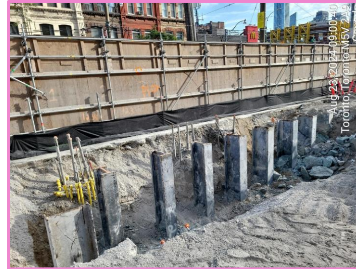
View of works in progress at the future South station site
