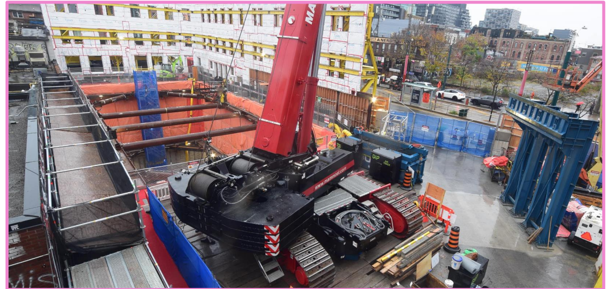
View of excavation work at the North site, October 2024
