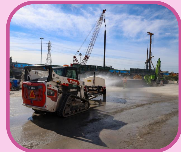
Ongoing water application
