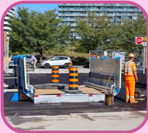
Wheel-wash installation
