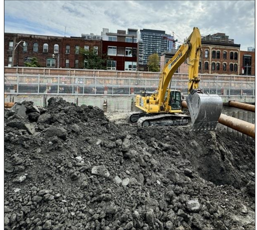
Example of shaft excavation and walers and struts installation.
