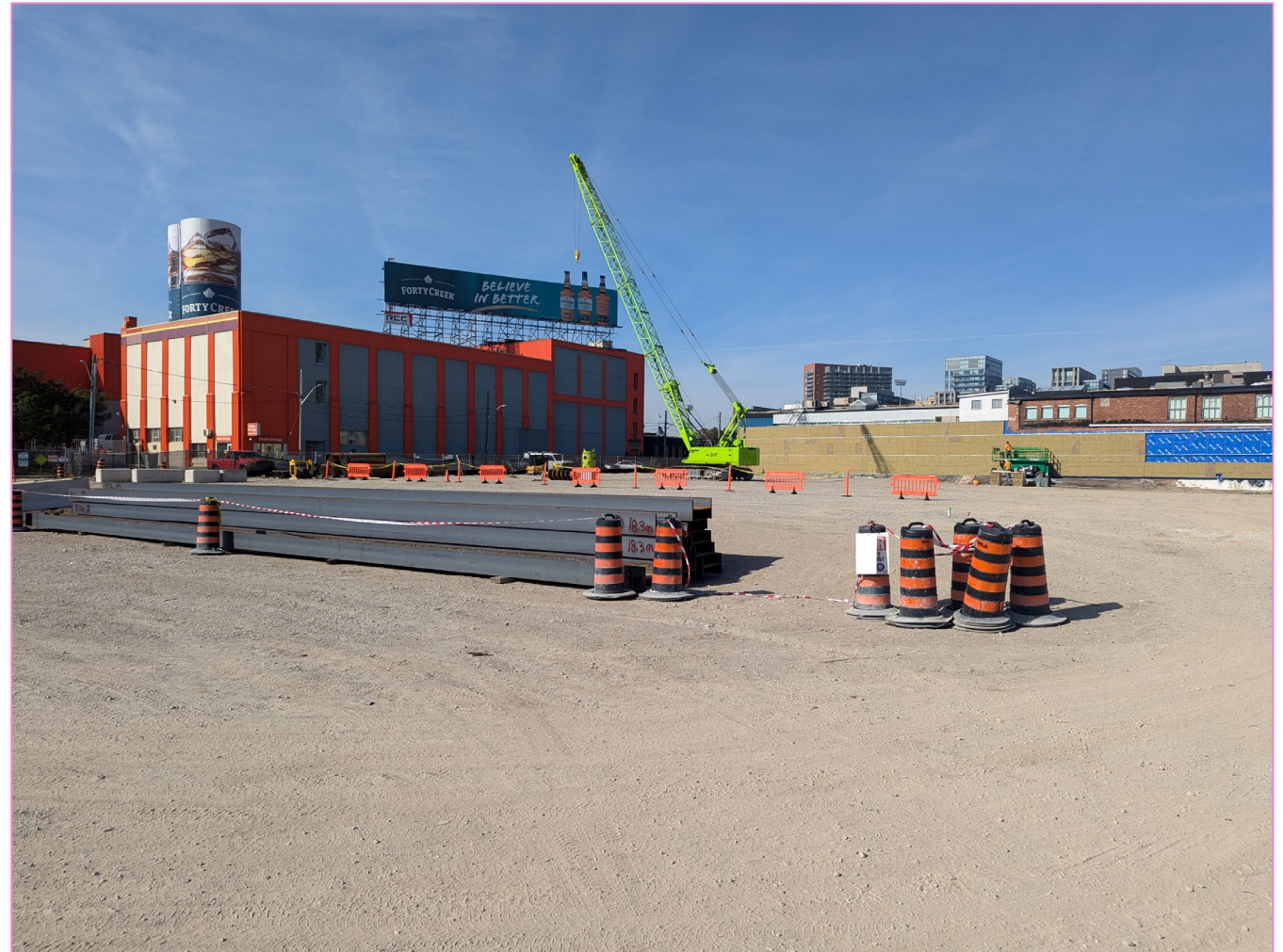
Graded land between Atlantic Avenue and Jefferson Avenue, looking south.
