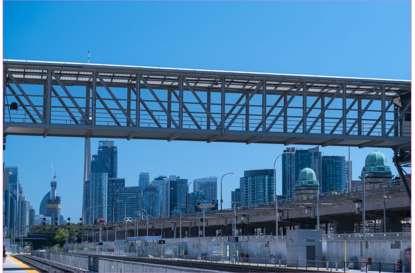
Exhibition Station temporary pedestrian bridge, looking east.
