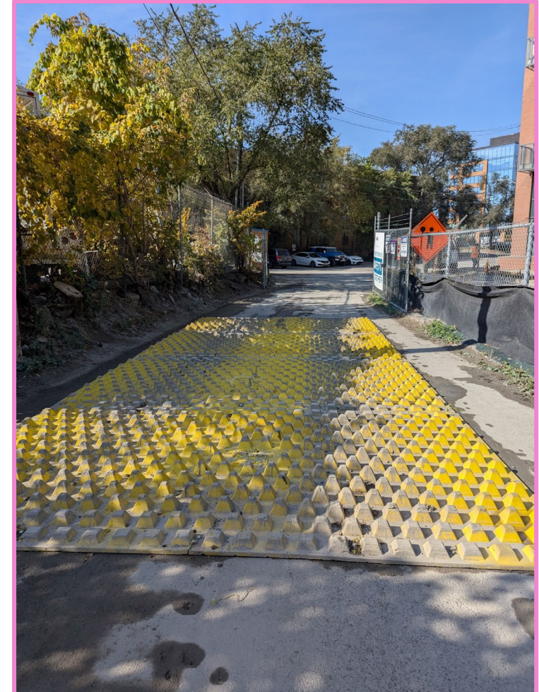
Wheel cleaning shaker mat, to ensure trucks do not bring mud and soil into city streets.
