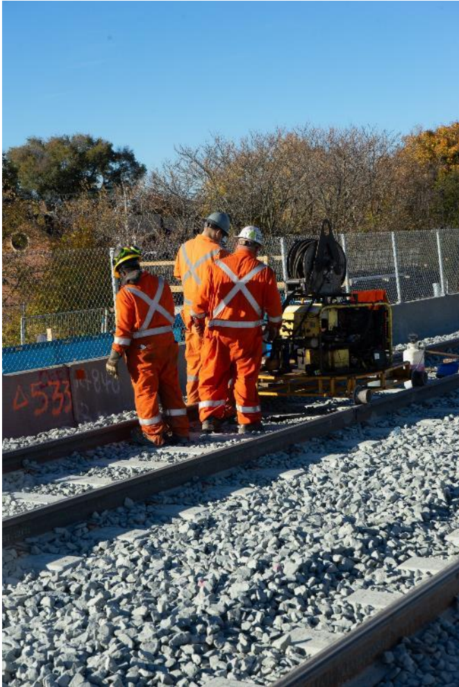
Workers welding tracks
