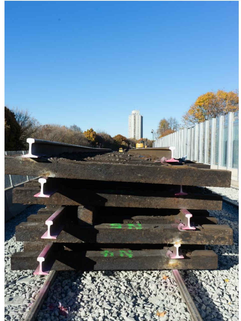
New tracks awaiting installation
