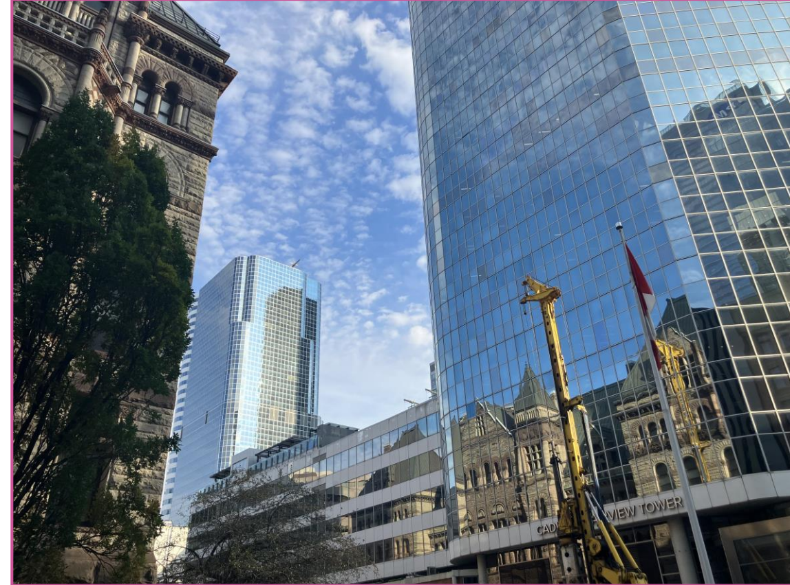
Piling Machine at the West site - November 2024
