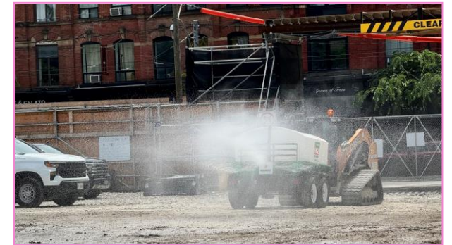
Example of dampening soils to suppress dust
