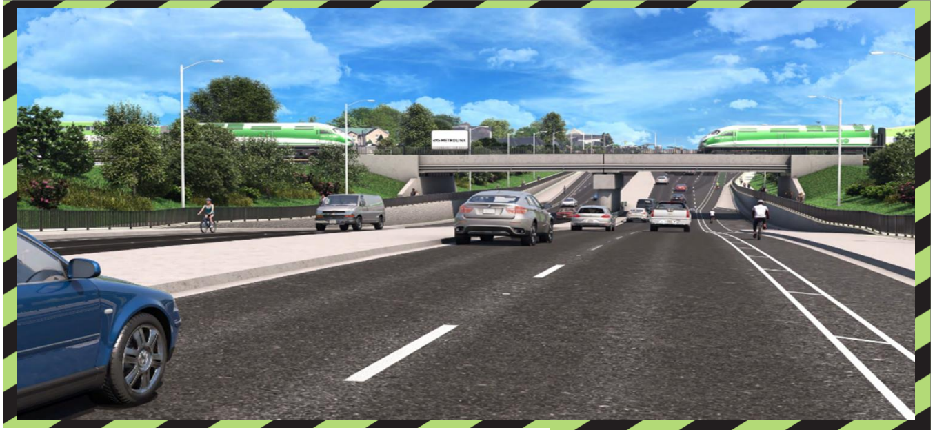
An image showing the Burloak Grade Separation and for illustrative purposes only.
