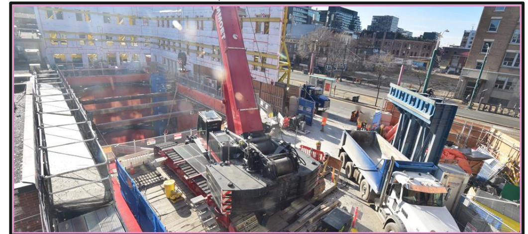
View of excavation at the future Queen-Spadina North station site.
