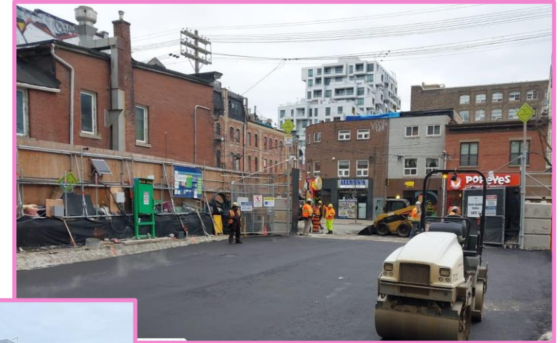
Paving completion at the South site
