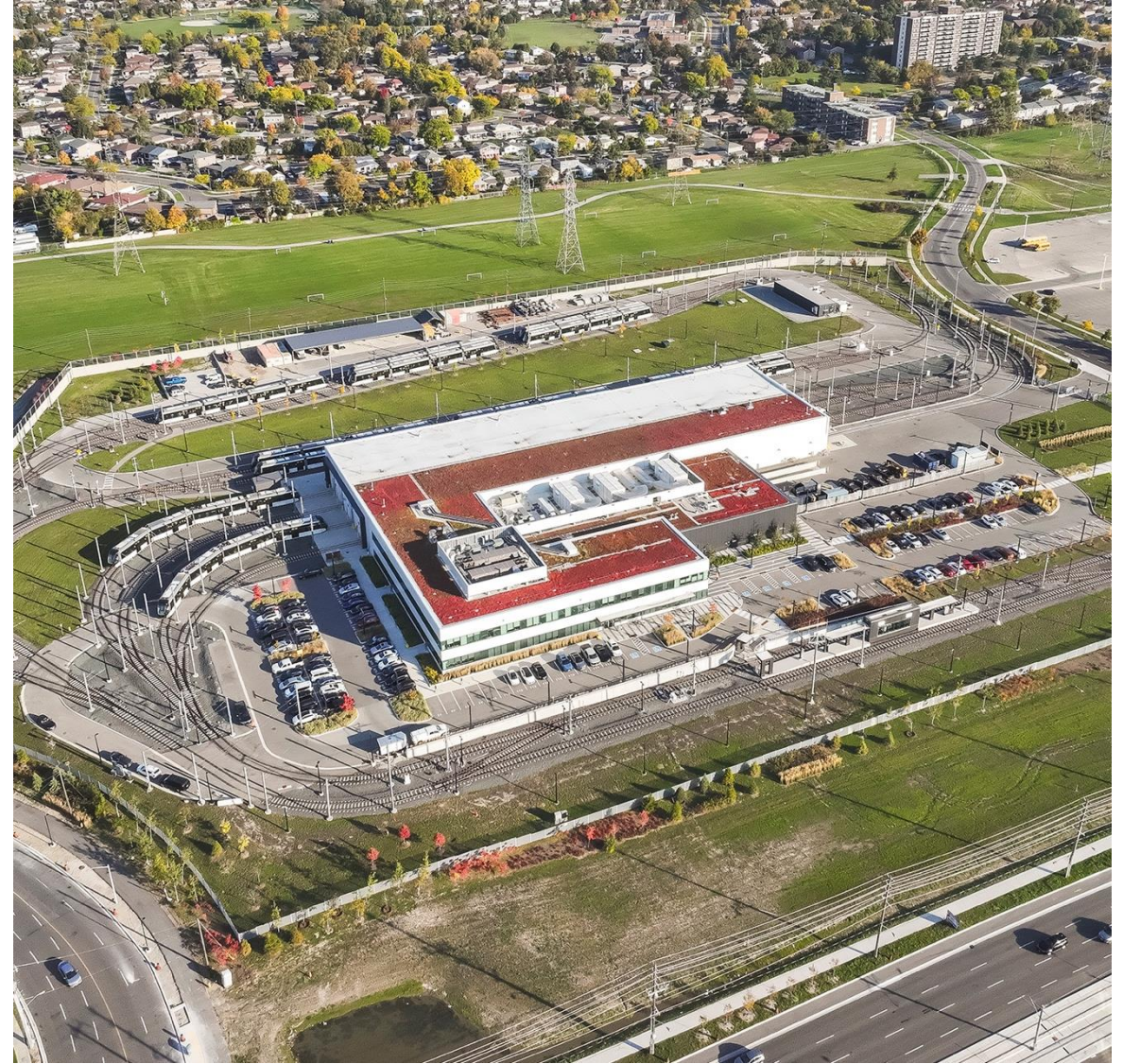
Photo: Maintenance and Storage Facility, northeast aerial view. 2024.10.21
