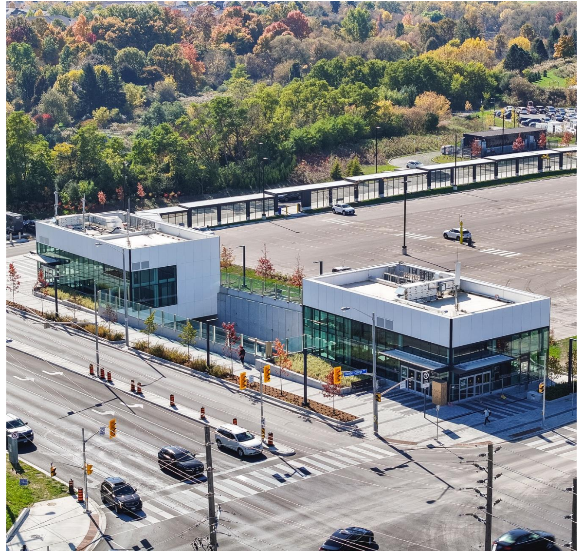
Photo: Humber College station, aerial view southwest. 2024.10.21
