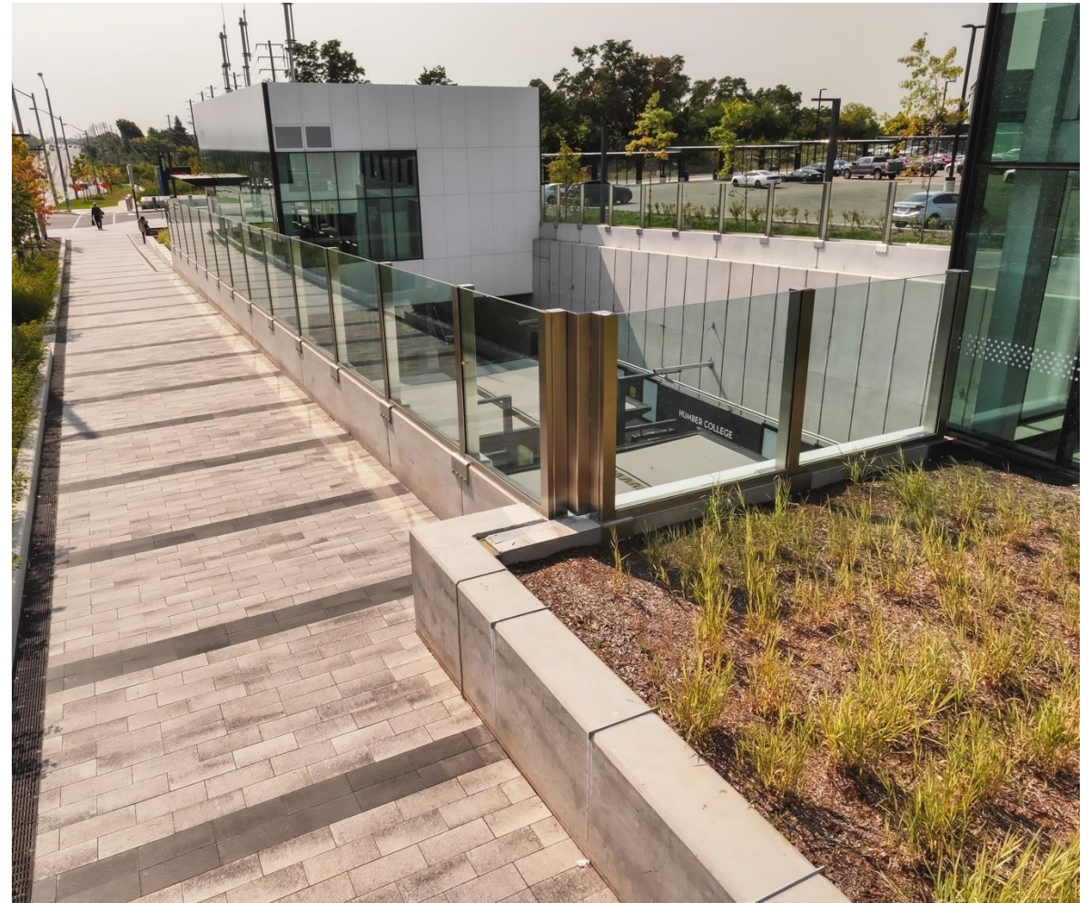
Photo: Humber College station exterior south building. 2024.10.01
