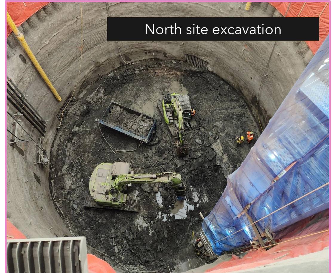
Looking down the excavation shaft, on the north site.
