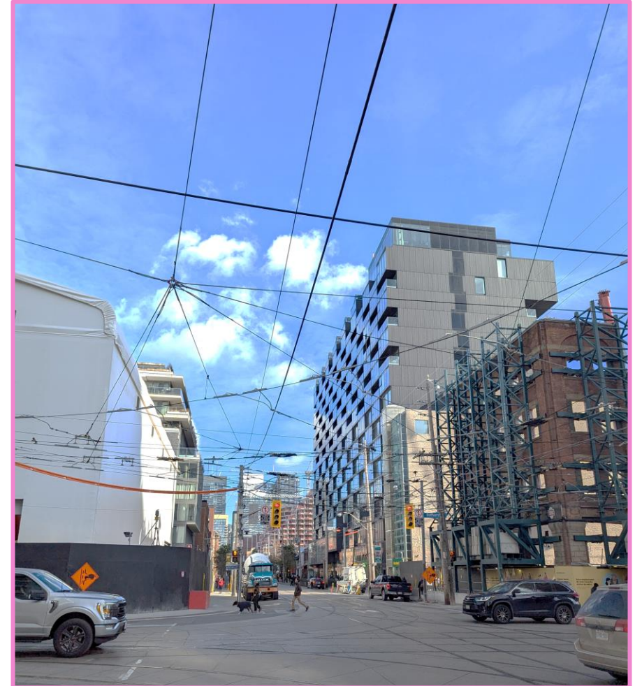
Construction work at the south site, facing Bathurst Street.
