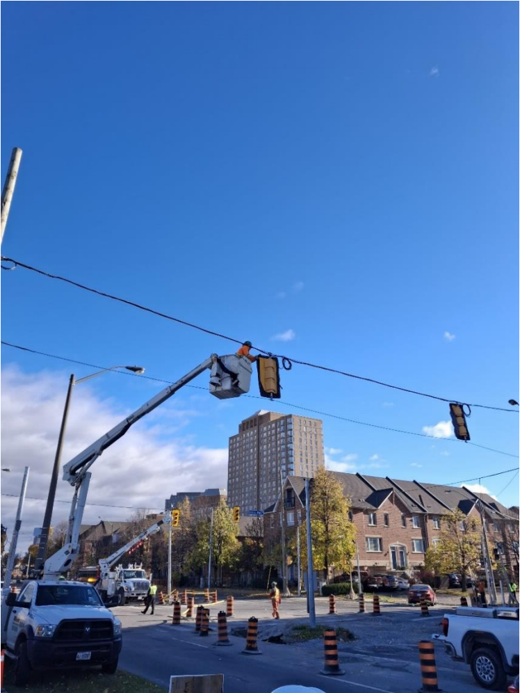
Temporary traffic signal installation
