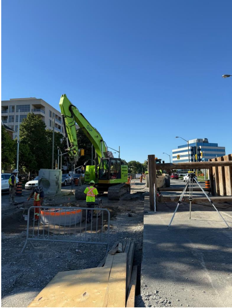
Median modifications Utility works
