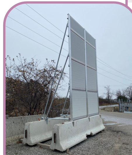
Noise barrier to be installed around piling at Queen bridge
