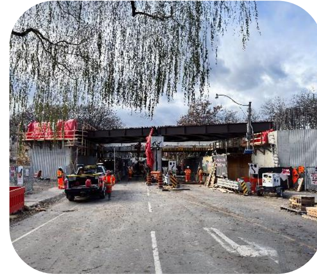
Installed second set of bridge girders at the Dundas bridge
