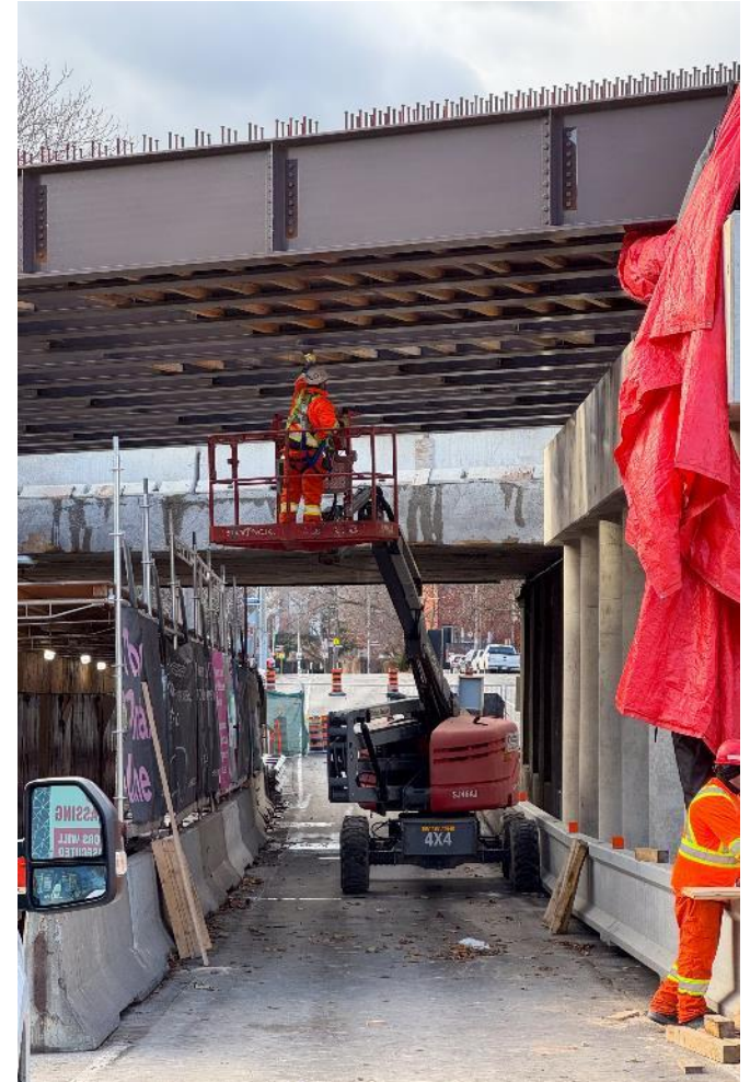
Preparing for pouring of concrete for new bridge deck
