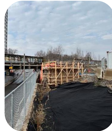
Completed Logan bridge abutment - 325m 3 of concrete poured
