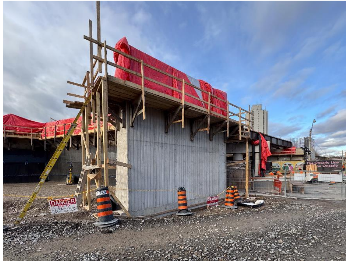
New bridge abutment along with new girders
