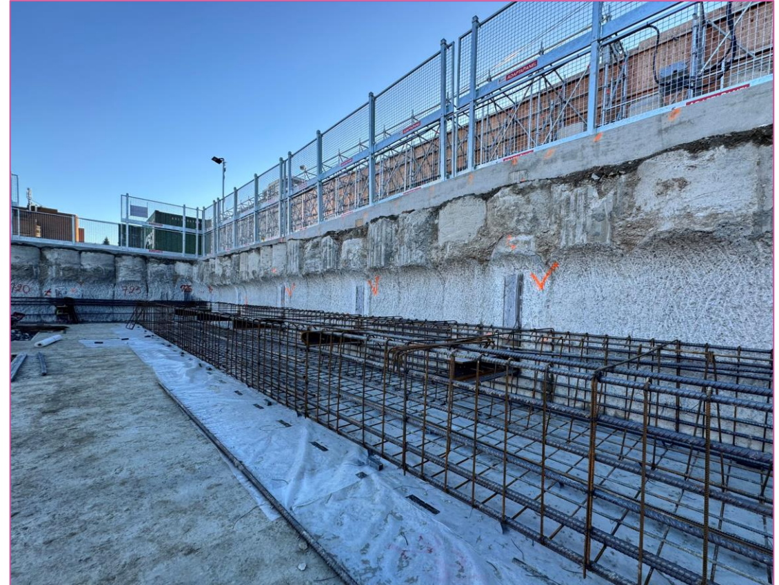
Rebar in preparation for formworks and concrete pour
