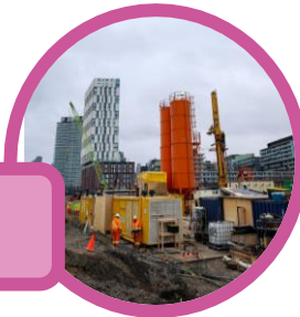
Jet Grout Preparation Plant
