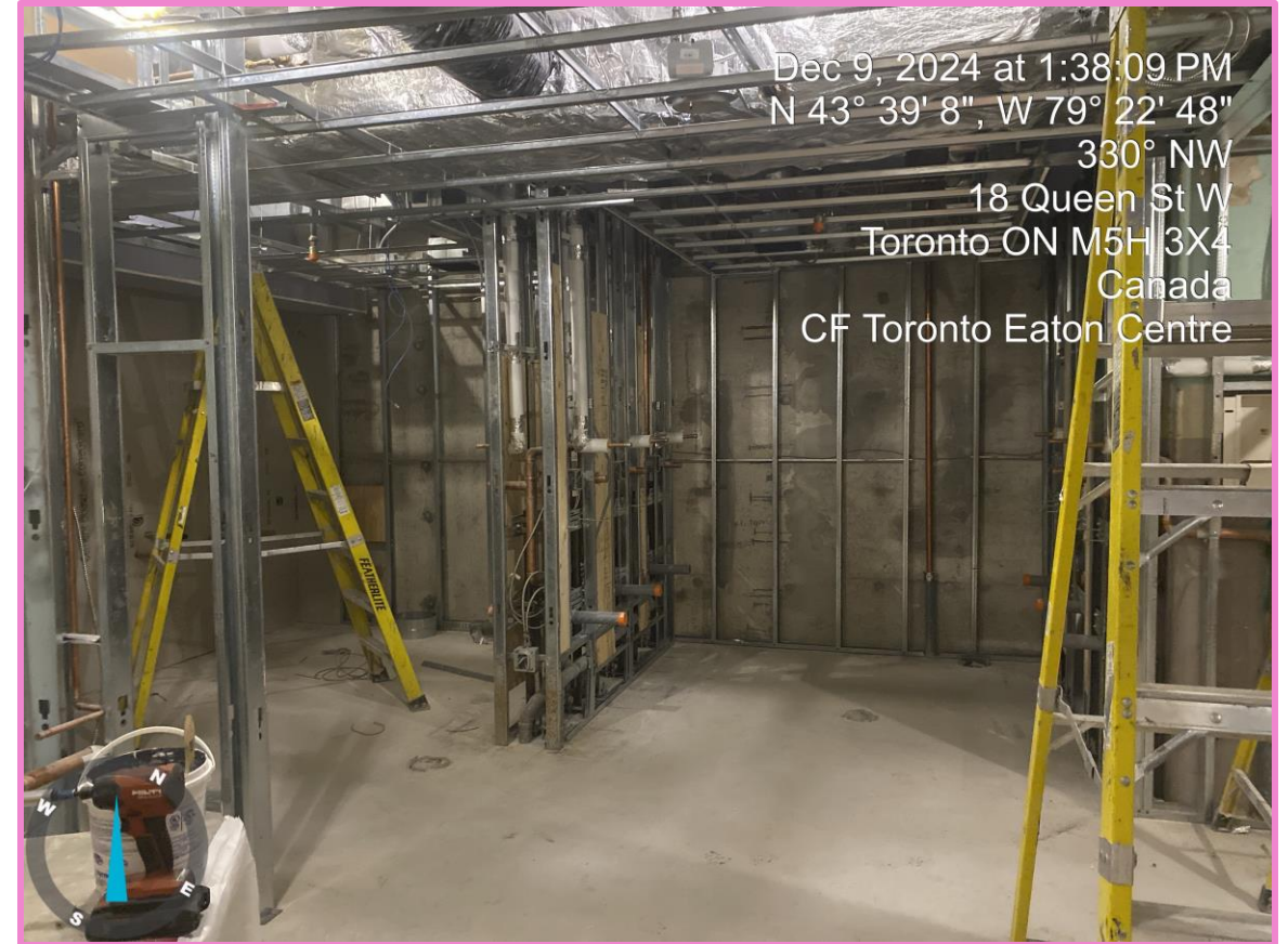
Mechanical Works in the Basement
