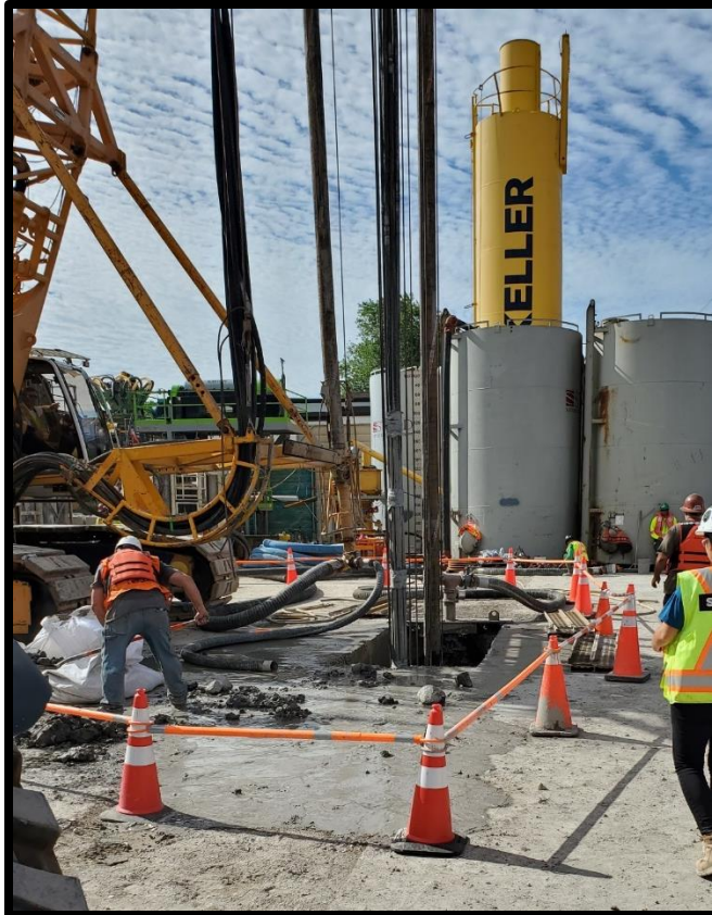
Excavating a panel with the hydromill
