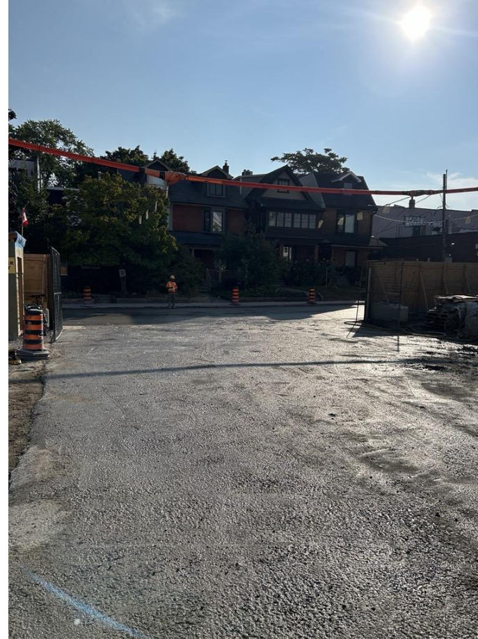
Concrete pad at the Eaton Gate
