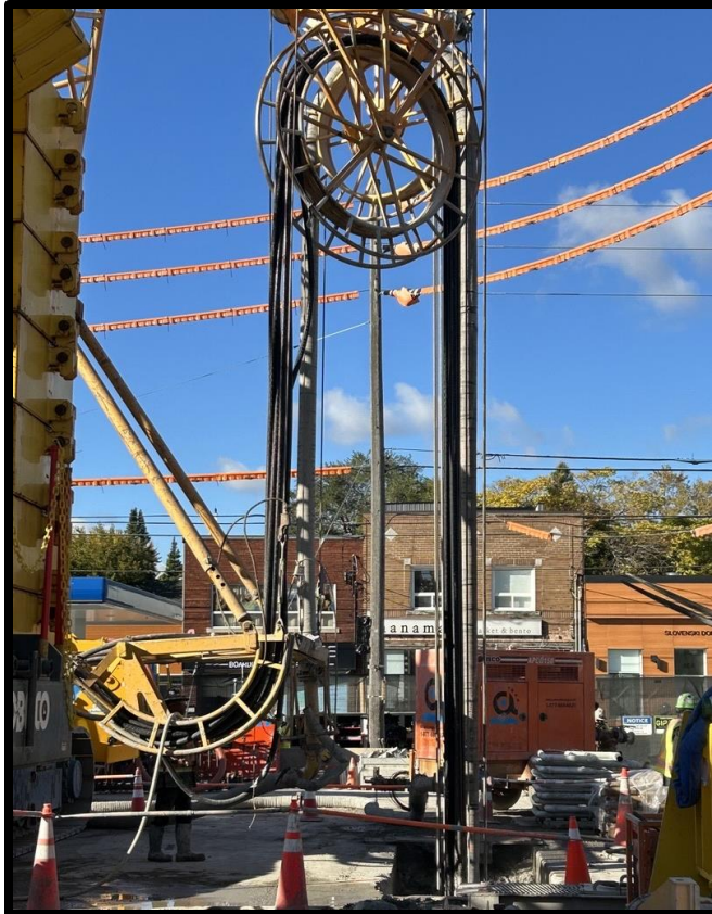
Excavating panel at Sammon
