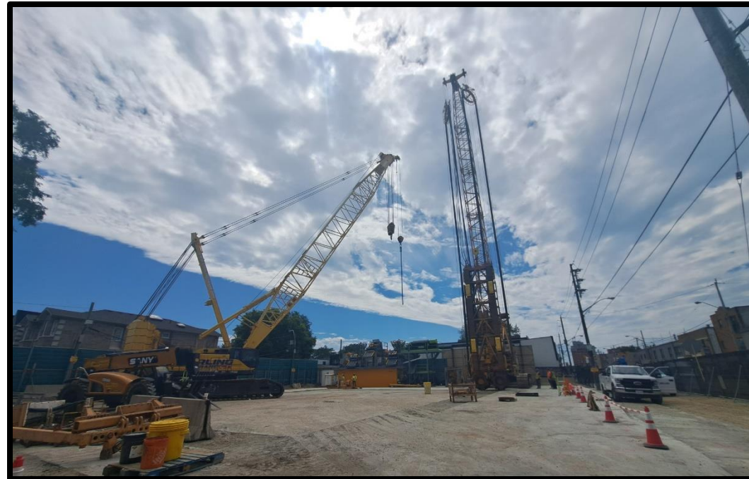
A crane and hydromill at the Sammon site
