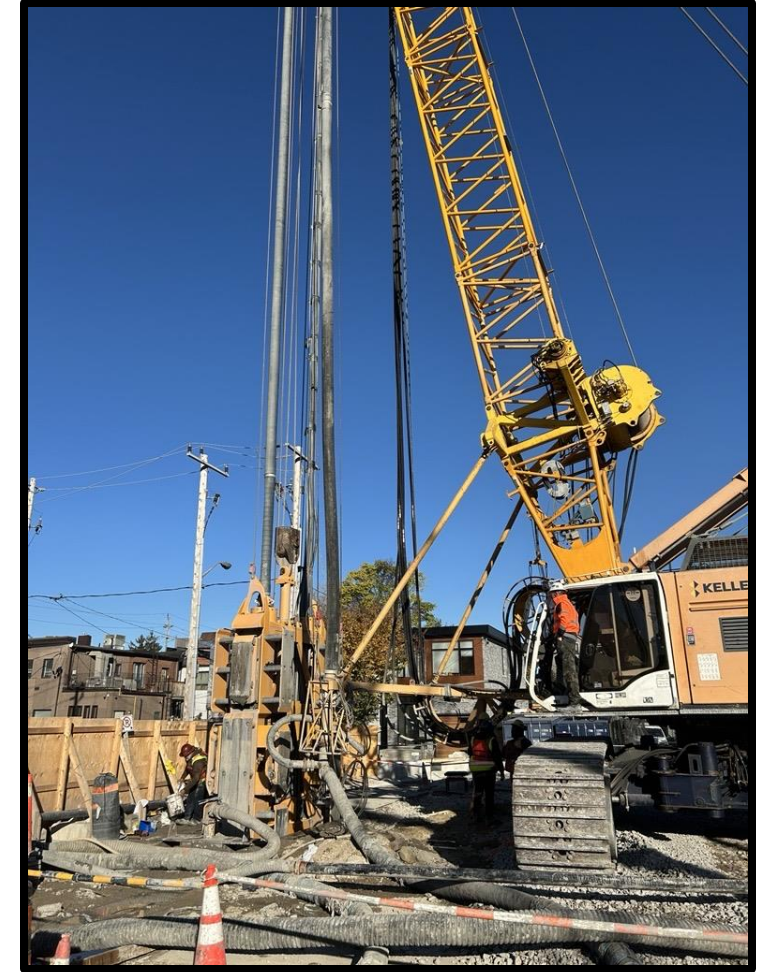
Excavating panel in Pape north shaft
