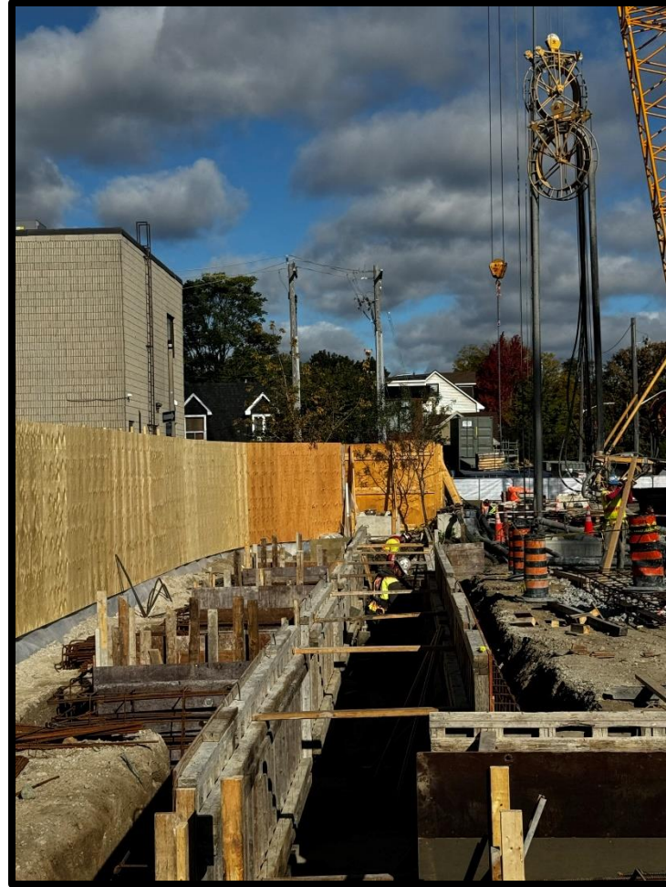
Building Pape north guidewall
