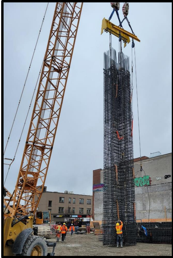
Lifting a rebar cage before inserting into excavated panel
