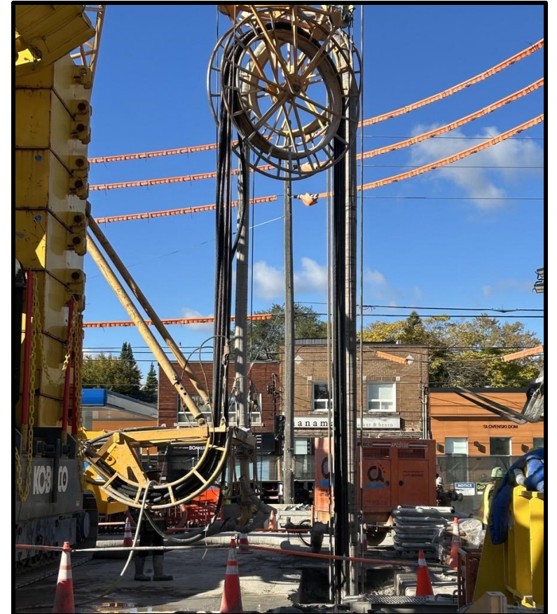
Excavating with the hydromill
