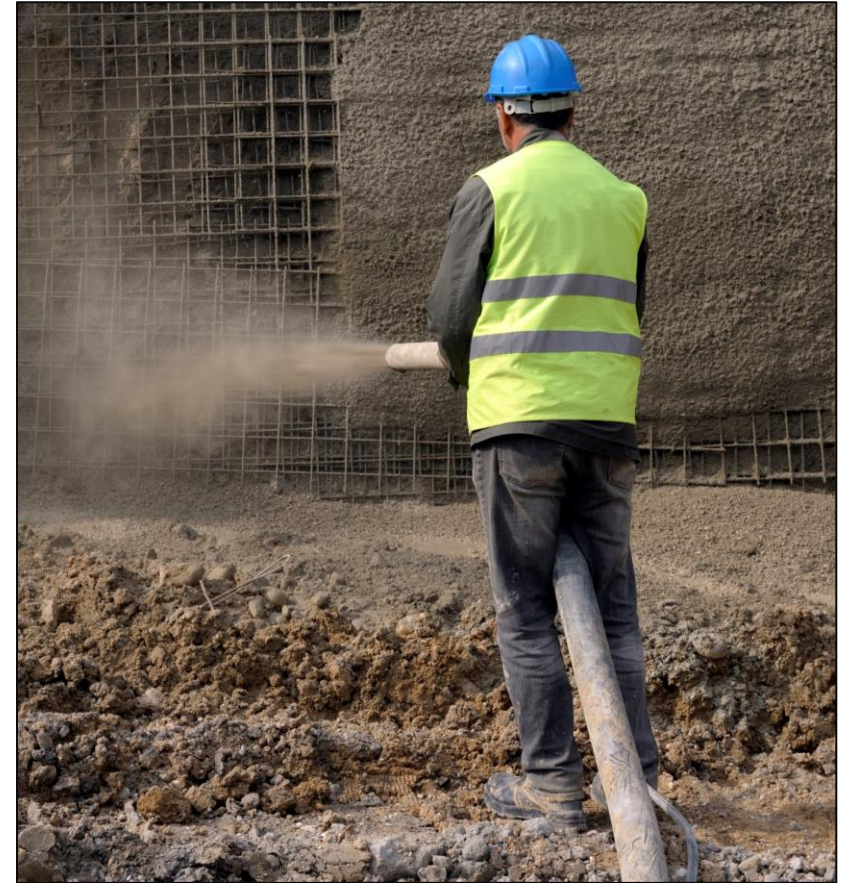
Example of shotcrete installation
