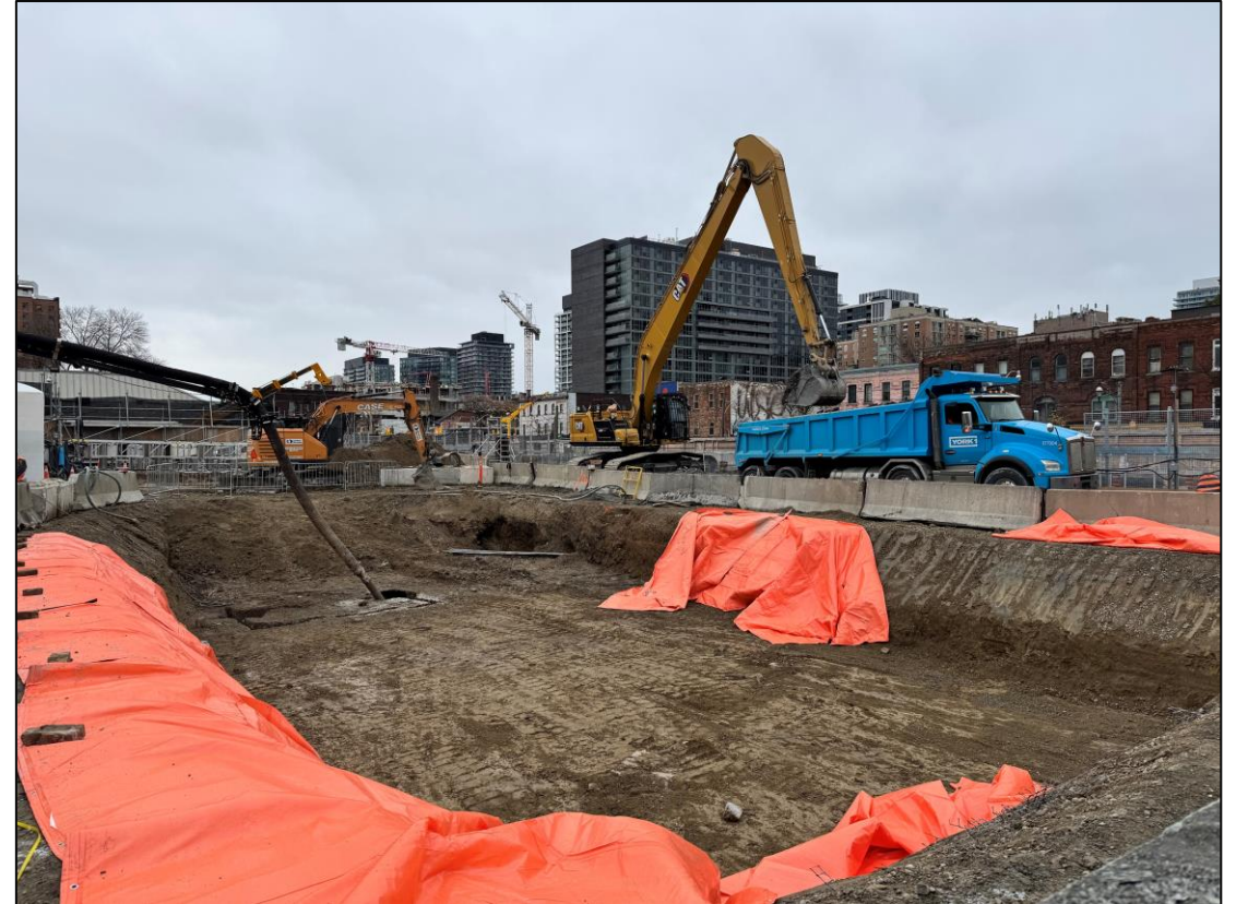
Tower crane platform in progress
