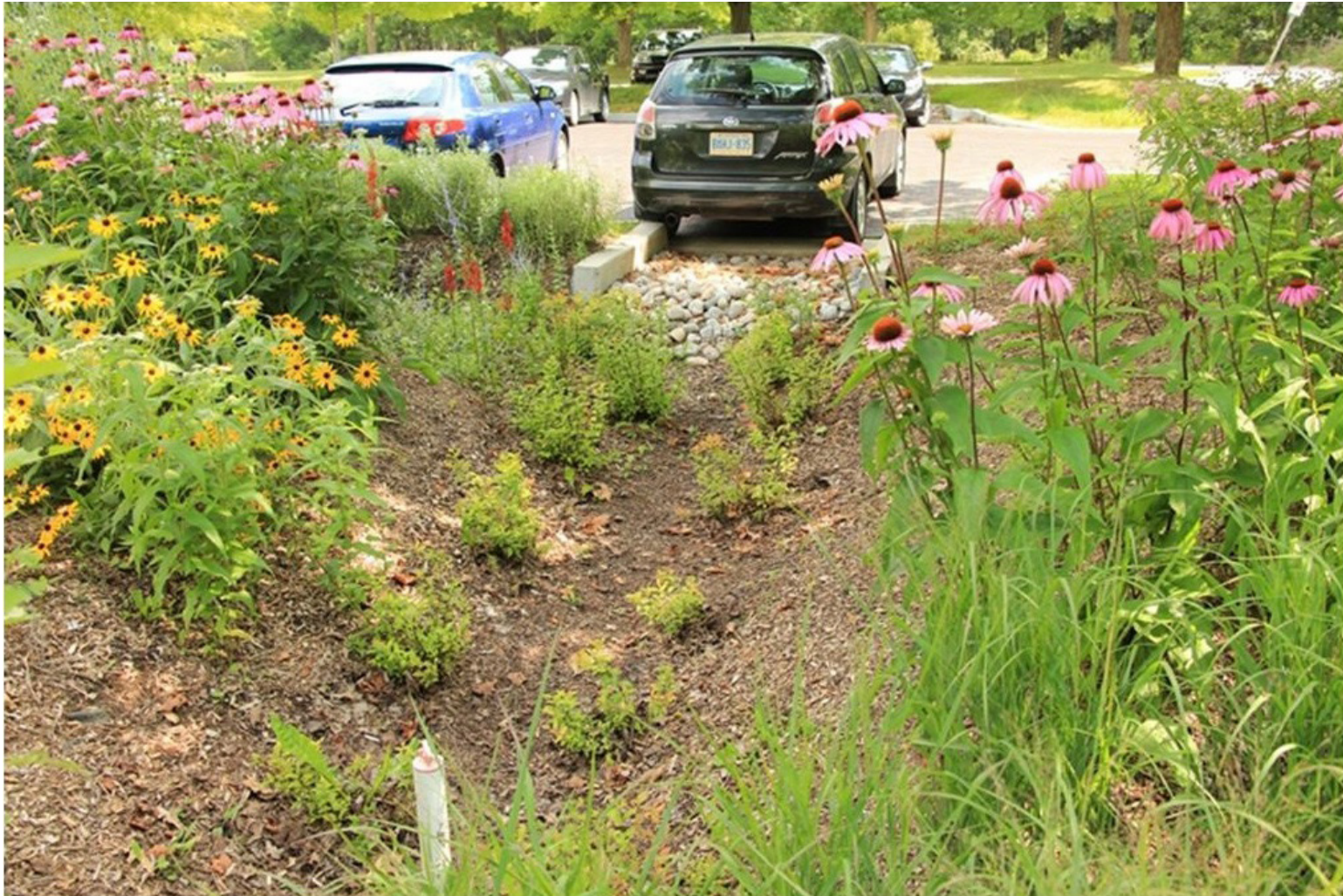
Bioretention Cell capturing and treating runoff from adjacent parking lot (Source: Sustainable Technologies)
