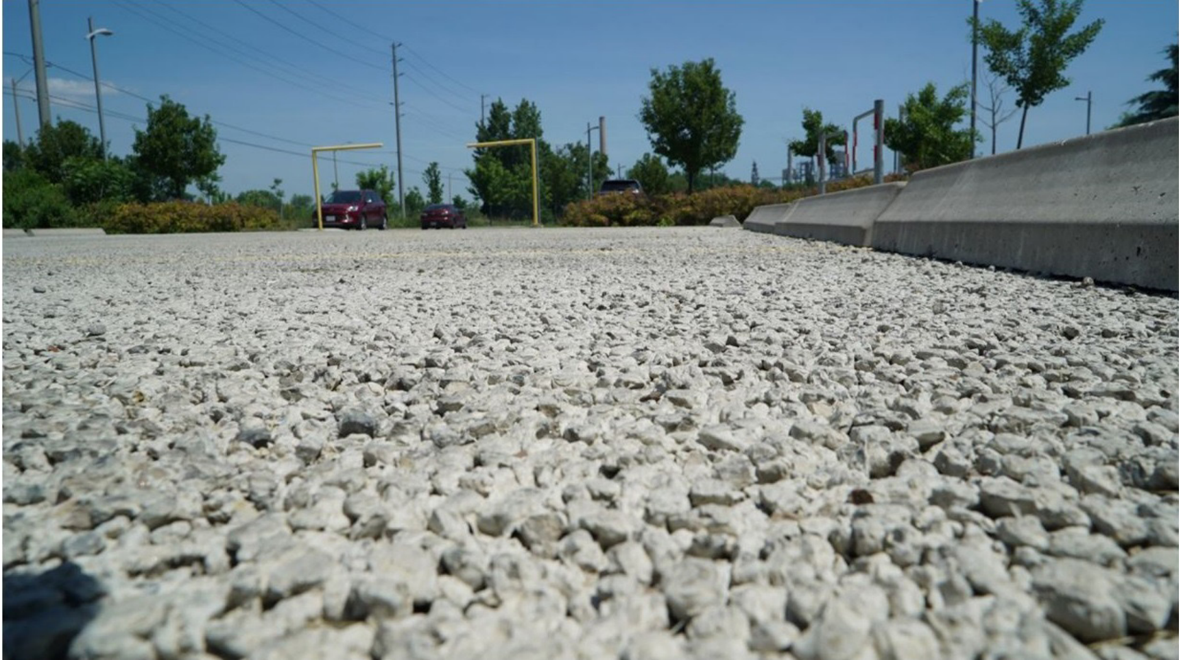
Permeable Concrete Paving at Lakeside Park, Mississauga (Source: wiki.sustainabletechnologies.ca )
