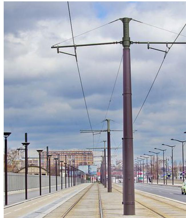
Figure 4-38: Overhead catenary system (OCS) poles
