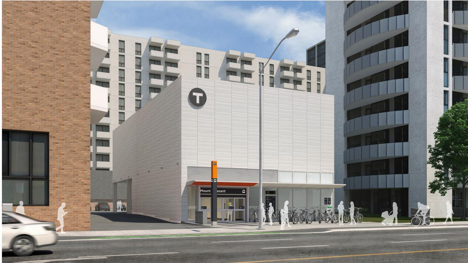
Figure 4-36: TPS on second floor integrated with a secondary entrance building
