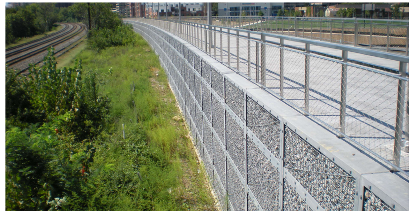
Figure 5-22: Guardrail and handrails
