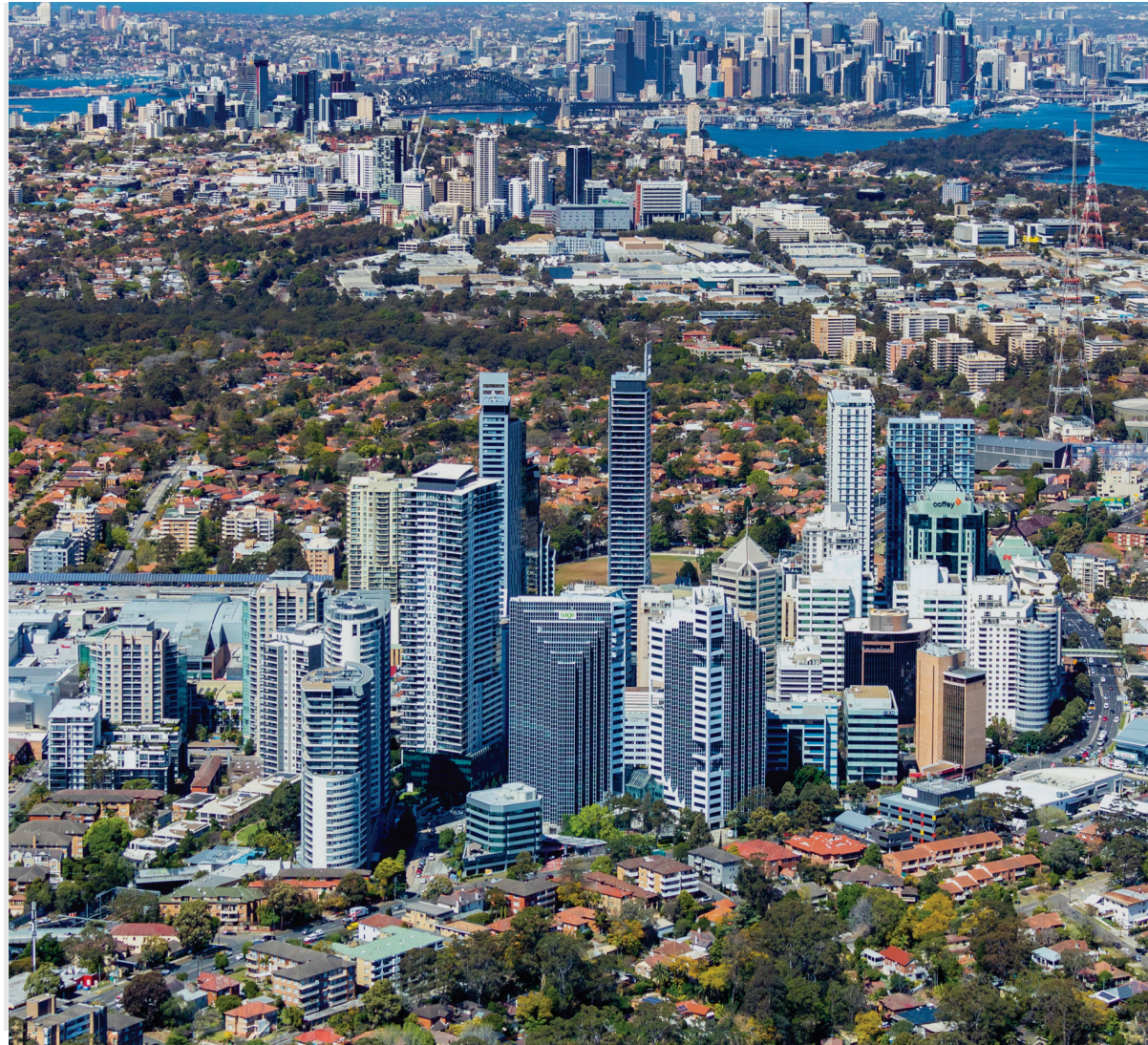
Figure 2: Chatswood Transport Interchange, Sydney Courtesy of Reddit.com
