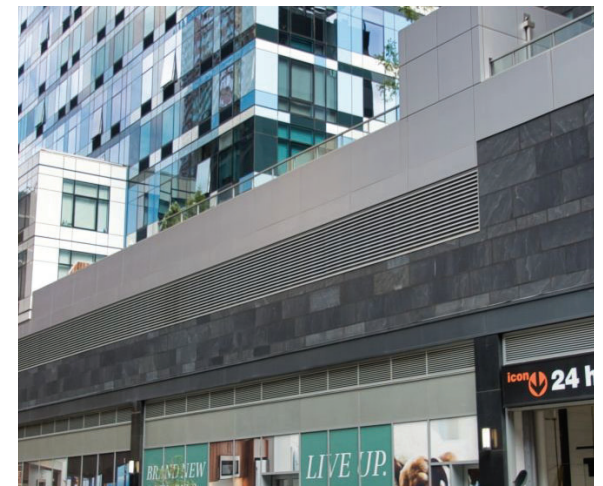
Figure 63: Jay St Metro Tech Station, New York Courtesy of Nicolas Janberg and structurae
