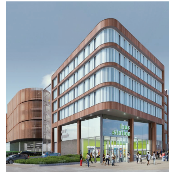
Figure 41: Broadmarsh Bus Station, Nottingham Courtesy of https://www.constructionenquirer.com
