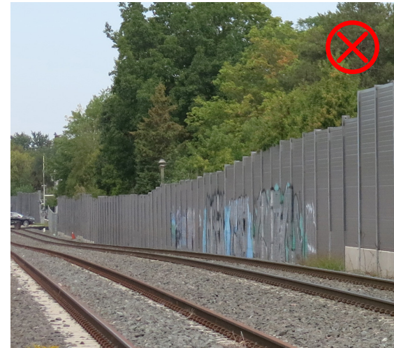
Figure 20: Noise barrier should not look like an accordion when responding to topographical changes
