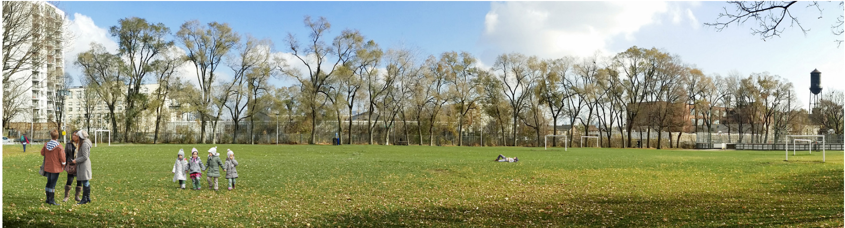
Figure 11: Davenport Diamond Grade Separation (pre-construction). Looking east across Cambell Park to the rail corridor prior to the construction of the elevated guideway. The view of the rail corridor from the park is partially concealed by a row of mature trees.
