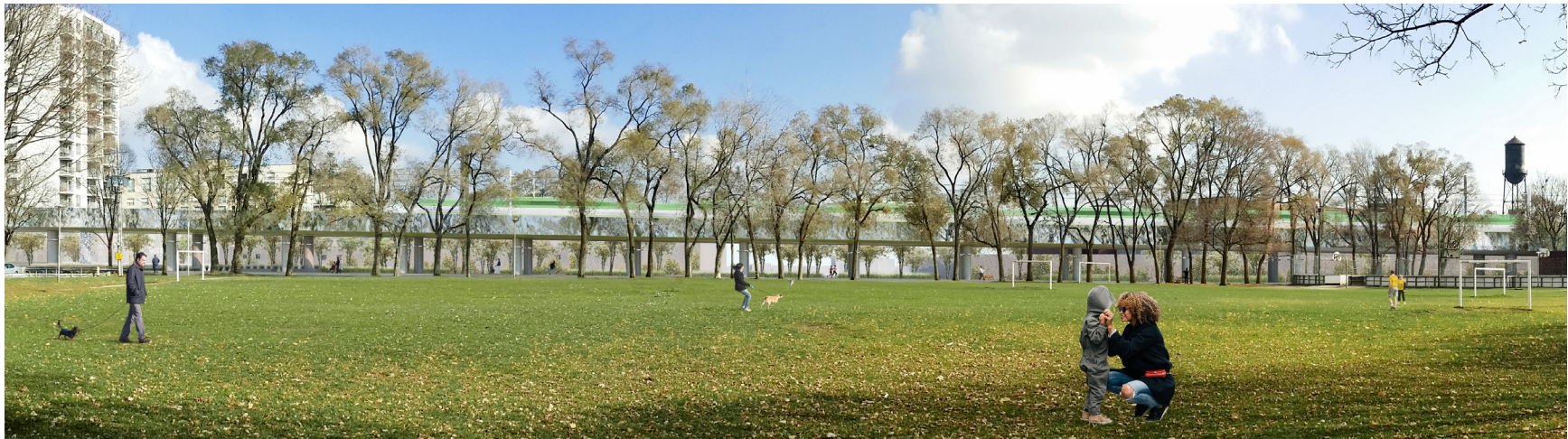
Figure 11: Davenport Diamond Grade Separation (post-construction). Looking east across Cambell Park after the construction of the elevated guideway. The view of the elevated guideway from the park is partially concealed by a row of mature trees while the views at-grade provide clear sight lines to the public landscaping and multi-use trail beyond.
