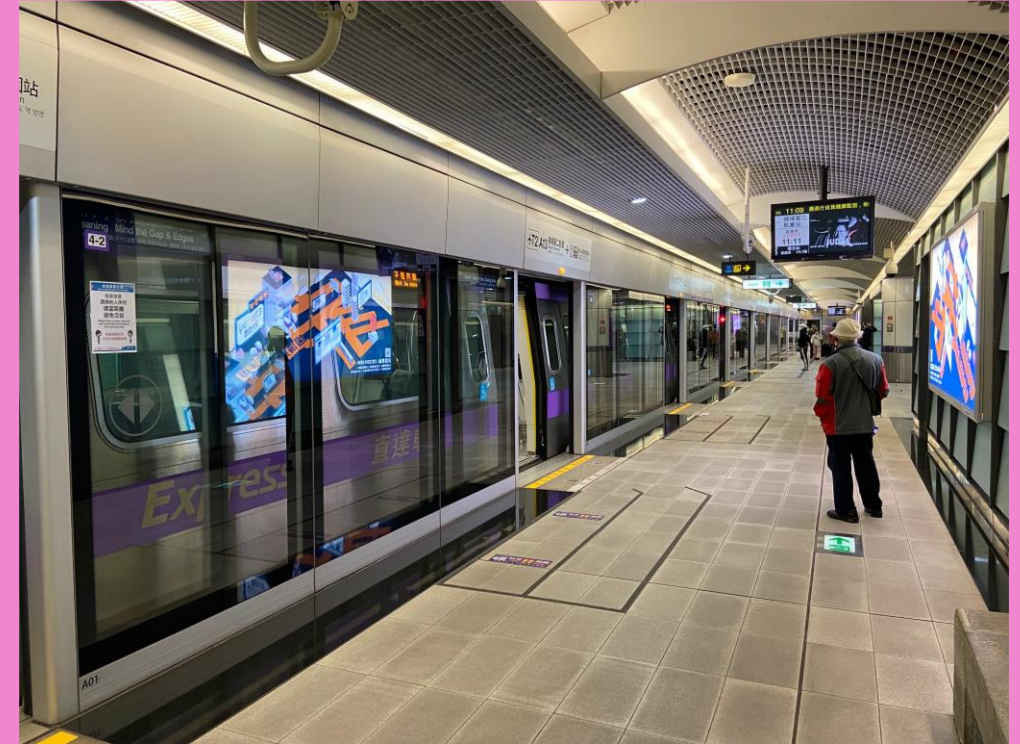
Example of platform screen doors currently in Chennai, India.
