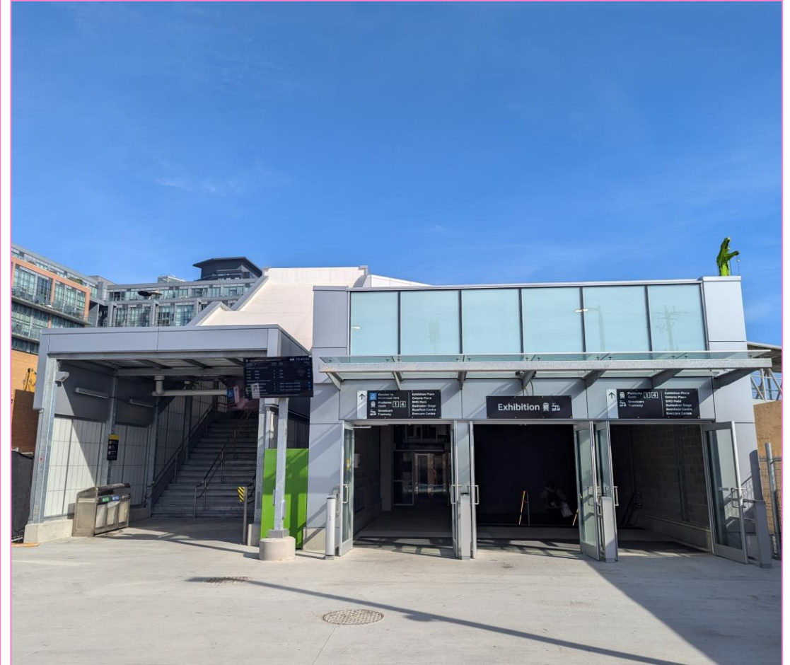
Right: Exhibition Station temporary pedestrian bridge, looking east.
