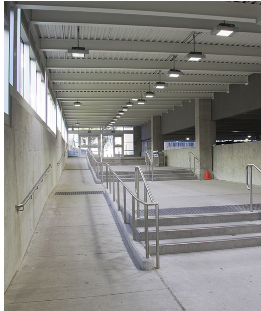
Figure 8: Typical Ramp - Ajax GO Station
