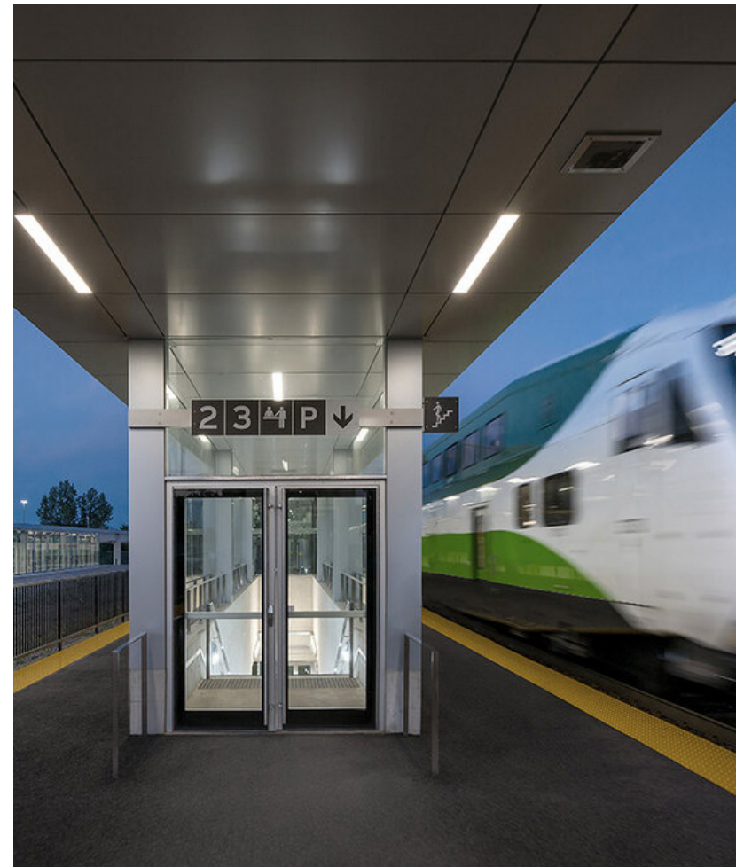
Figure 1: Typical Platform - Guildwood GO Station
