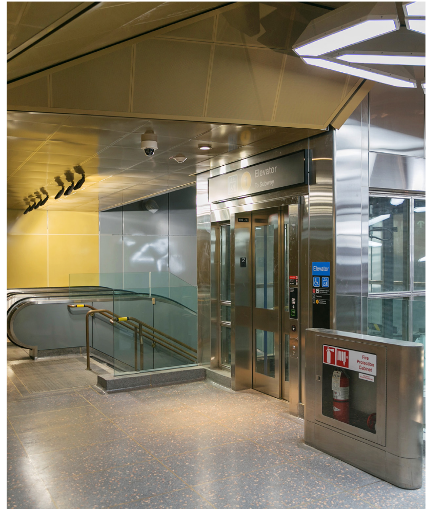
Figure 7: Typical Elevator - TTC Pioneer Village
