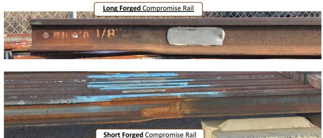
**Note:** "Long Forged" Compromise rails have a forged section of approximately twentytwo inches. They can be identified by having only a short length of the compromise rail in the smaller rail section. "Short Forged" compromise rails have rail weights that are typically evenly split between the two rail sizes and can continue to be used.
