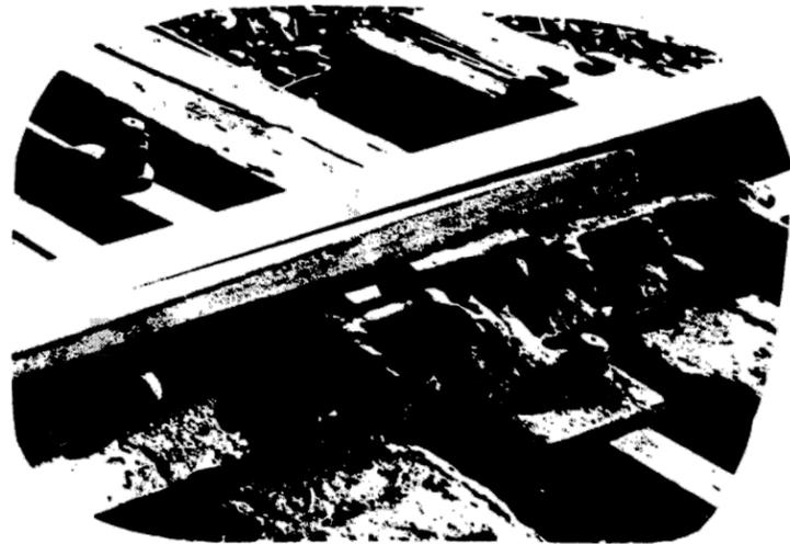
A PROPER INSTALLATION FOR A SWITCH POINT LOCK IS ON THE SECOND HEAD BLOCK TIE, BETWEEN THE CONNECTING ROD AND THIS TIE, AS SHOWN. THE HAND LEVER OF THE "CLOSED SWITCH" SWITCH STAND MUST ALSO BE OVER THIS TIE. IF THE HAND LEVER IS OVER THE FIRST TIE IN THE CLOSED POSITION, SUGGEST CHANGING THE POSITION OF THE HANDLE ONLY TO ALLOW HAND LEVER TO REST OVER SECOND TIE IN THE CLOSED SWITCH POSITION.
