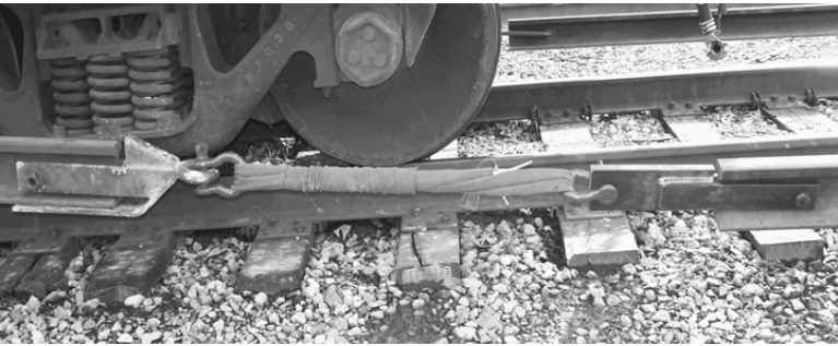
Figure 11. End of one rail connected to the beginning of another being unloaded
