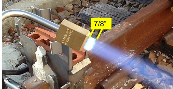
Figure 10-21: Oxygen-Propane Proper Feathered Flame Length
