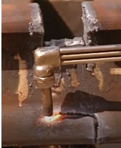
Figure 8-2: Torch Cutting the Head and Base
