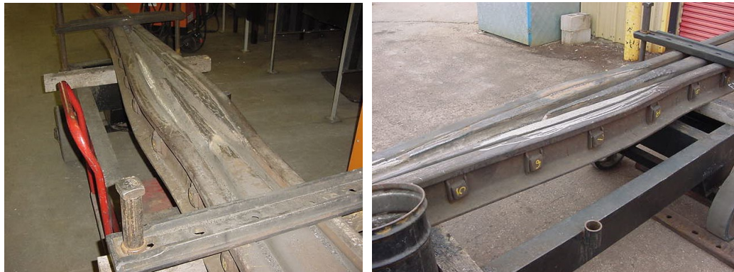
Figure 14-7: Frogs Being Repaired in a Strongback Jig Courtesy CN Training
