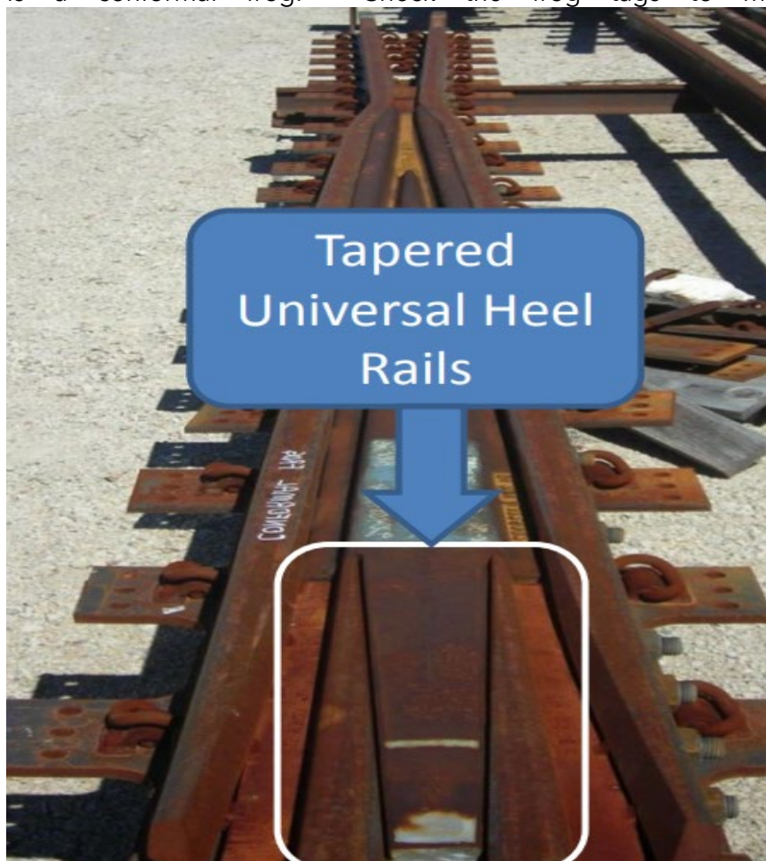
Figure 6-39: Tapered Universal Heel Rails of Conformal HP Frog
