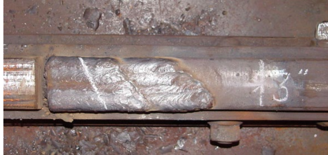
Figure 7-7: Weld Area and Post-Heat Measurement Courtesy CN Training
