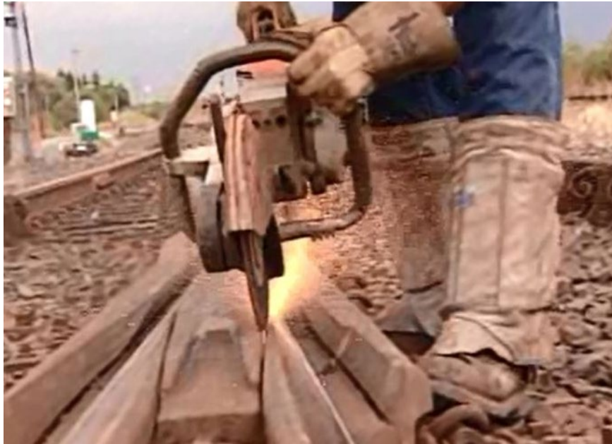
Figure 6-21: Slotting Frog Heel Rail Contact Mating Surface
