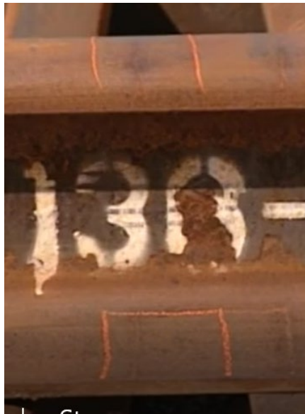
Figure 8-1: Marking the Rail for Torch Cutting
