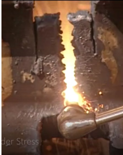
Figure 8-3: Cutting the Web with a Weave Pattern
