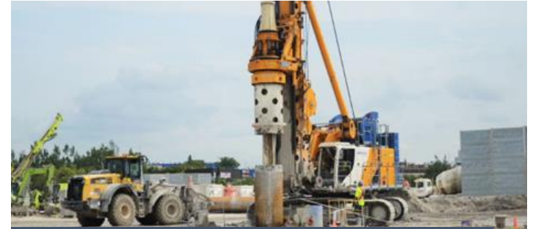
Scarborough Subway Extension Piling Work.
