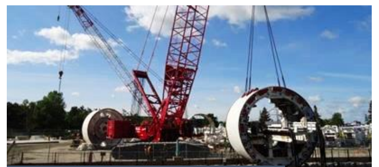
Lowering TBM cutterhead at YYSSE.
