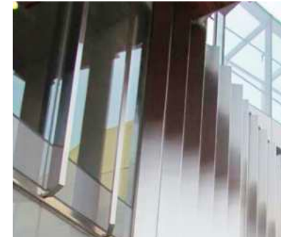
FACADE SUN BAFFLES (FB1) Material: Aluminum baffles Colour: Light grey Location: Exterior facade with southern exposure
