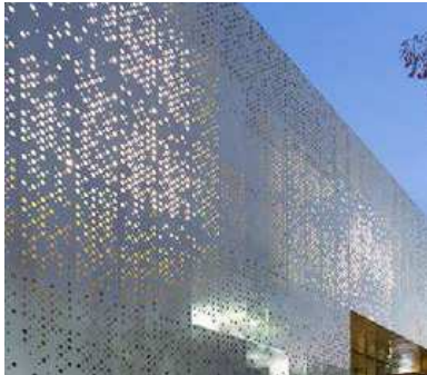
EXTERIOR SHADING SYSTEM (ES1) Material: Perforated aluminum panels Colour: White Pattern: Variable Location: Exterior cladding on Station
