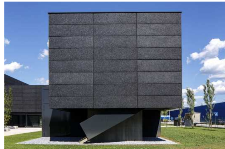
Figure 4-26: Precedent image demonstrating use of opaque wall system cladding on an EEB that has been integrated with other back of house elements and clad in the same materials for an integrated architectural expression. Faber Headquarters, Battipaglia, Italy, by Geza. Image Courtesy Massimo Crivellari
