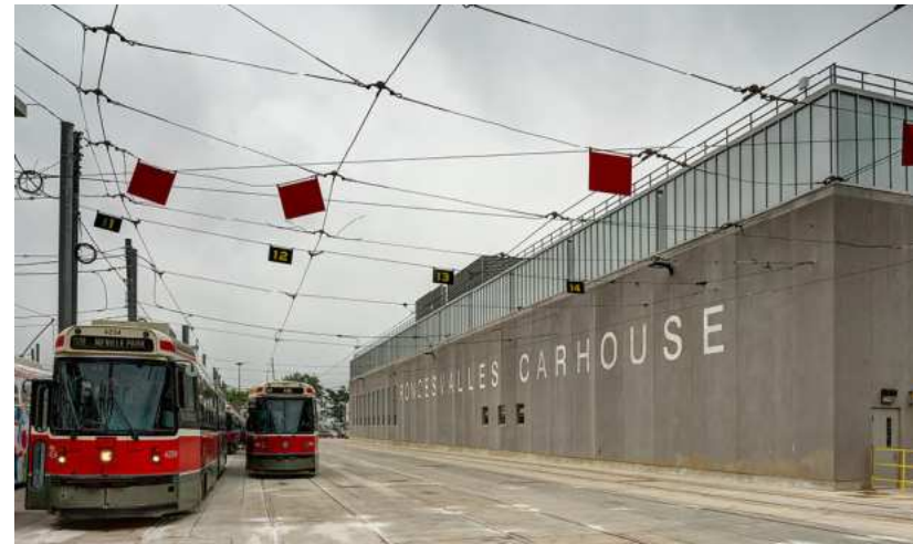
Figure 4-58: Precedent image demonstrating the use of opaque wall system cladding in a modular fashion for a larger maintenance storage facility (MSF) including an approach for ample natural light. TTC Roncesvalles Carhouse, Toronto, by Strasman Architects Inc.
