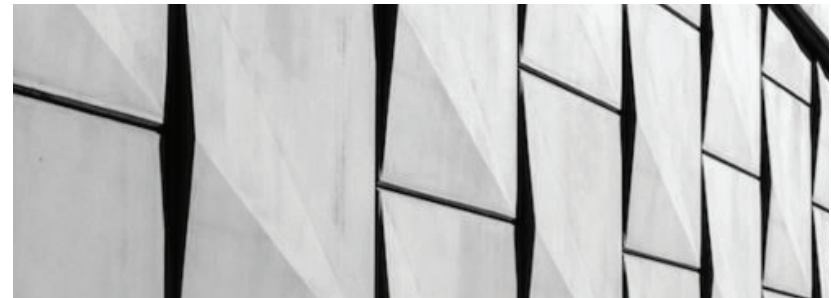
Figure 3-59b: Elevated Sound Barrier - Concrete
