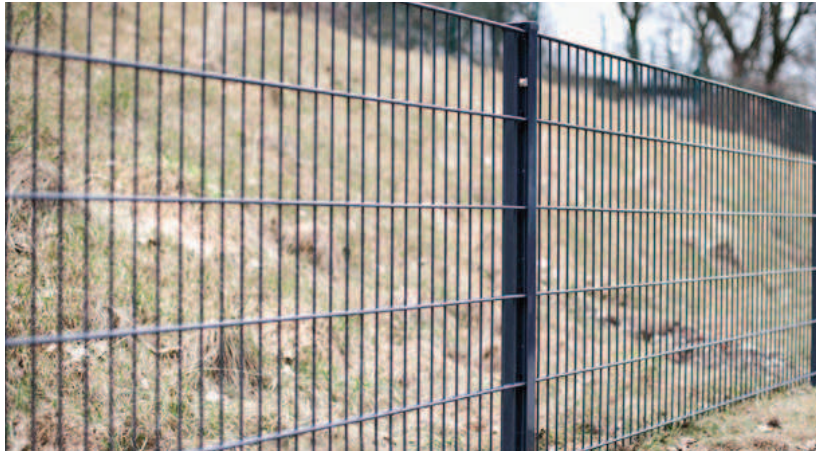
Figure 3-55a: Wire Mesh Fence
