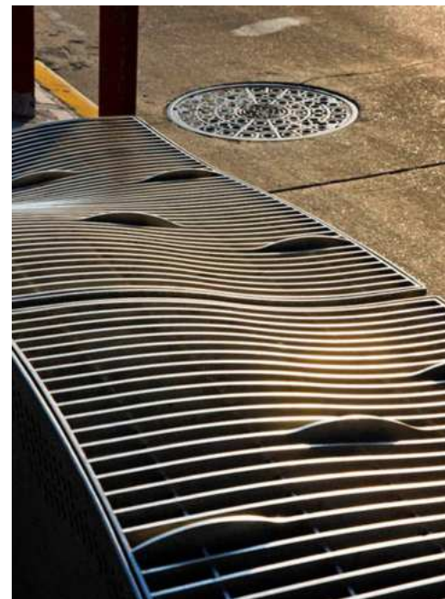
Figure 3-62: Tunnel Ventilation Shafts with Integrated Seating
