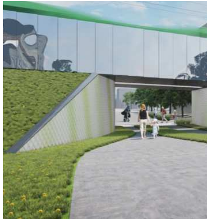
Figure 3-57: Retaining Wall - Coloured and pattern concrete
