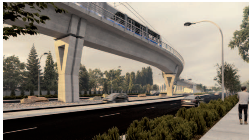
Figures 4-53 to 4-54: Precedent images demonstrating minimizing the impact of an elevated guideway in the public realm through tapering of elements, continuity of horizontal lines, concealing of clutter, an maximizing slope of guideway at portals to demonstrably minimize obstructions at grade. Valley Line LRT, Edmonton, Alberta, by Dialog.
