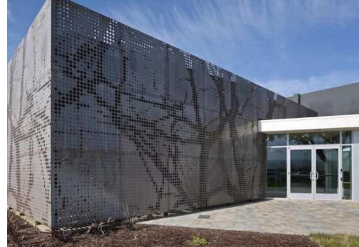
Figure 4-25: Precedent image demonstrating use of perforated metal cladding with creative perforation patterns on an EEB in the public realm. One Workplace, Santa Clara, California, by Design Blitz. Image Courtesy © Bruce Damonte
