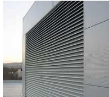
LOUVERS (LV1) Material: Aluminum slats Colour: To match building facade Location: Exterior stations, EEB's, Ancillary Buildings
