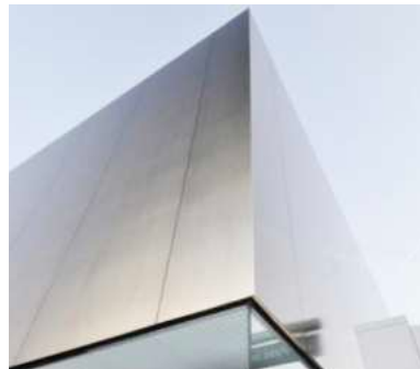
OPAQUE CLADDING (EW1B) Material: Prefinished composite metal panels Colour: Light grey Finish: Smooth Location: Exterior cladding stations
