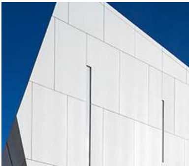
OPAQUE CLADDING (EW1A) Material: High performance porcelain/ceramic panels Colour: Light grey Finish: Matte Location: Exterior cladding stations
