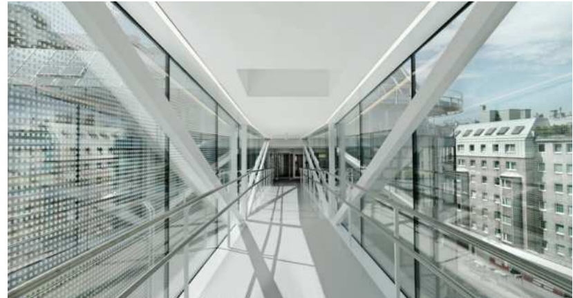
Figure 4-52: Precedent image demonstrating a pedestrian bridge using ceramic frit as a shading strategy. Bridge in Vienna, Austria, by SOLID architecture. Image Courtesy Günter Kresser
