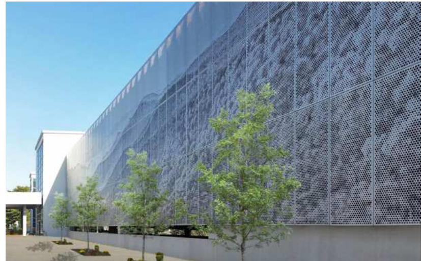
Figure 4-16: Precedent image demonstrating use of perforated metal cladding as an exterior feature element, creating a site specific station identity through printing of imagery. Ashville Regional Airport, Fletcher, North Carolina by Gresham Smith and Partners
