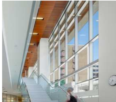
GLASS CURTAIN WALL (CW) Material: Glazed aluminum wall system Colour: Light grey Location: Main entry/exits
