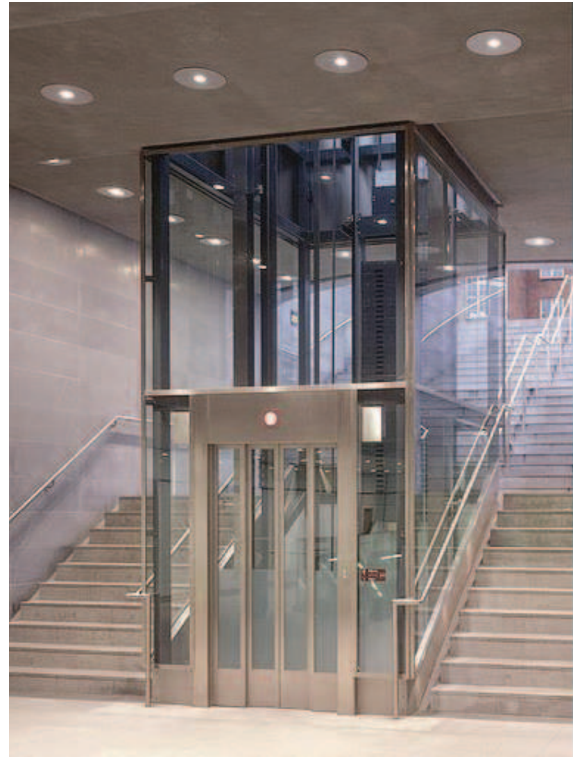
Figure 4-32: Precedent image demonstrating the transparency of materials required for subway station elevators. Copenhagen Metro, Cityringen, Denmark. Image Courtesy Peter Bartonbach @ Bartenbach GmbH
