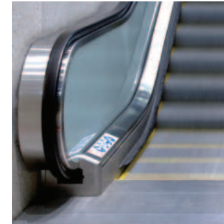
Figure 4-33: Precedent image demonstrating stainless steel enclosure and frosted glass balustrade adjacent to wall.
