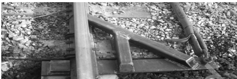
Figure 4. Rail grip used to anchor rail to track structure
