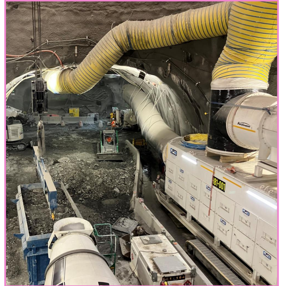
“Duduster” machine keeping the air clean in the station cavern.
