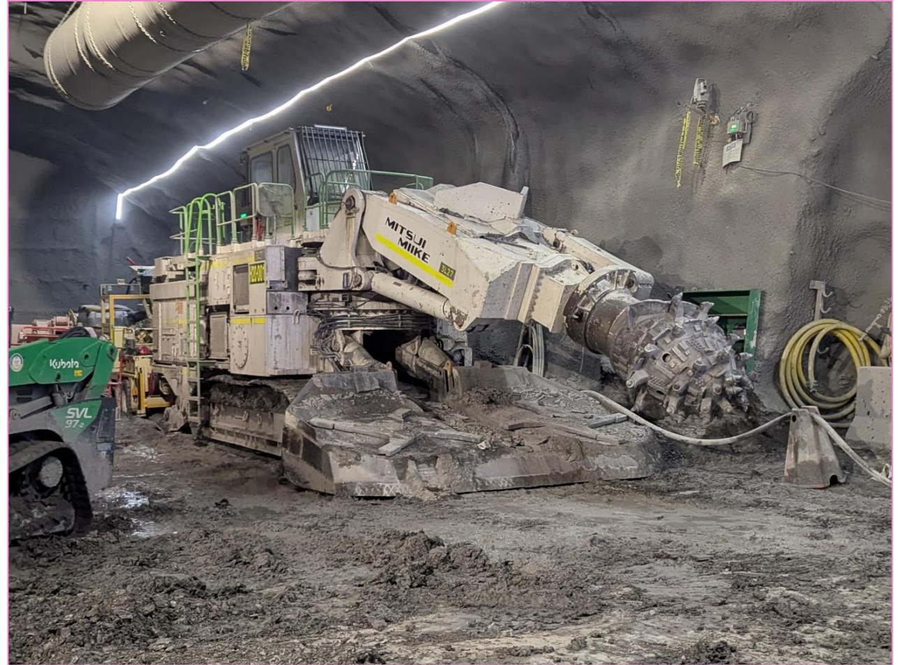
Roadheader machine in use at King-Bathurst
