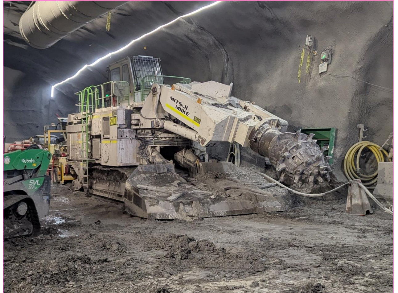
Roadheader machine in use at King-Bathurst site
