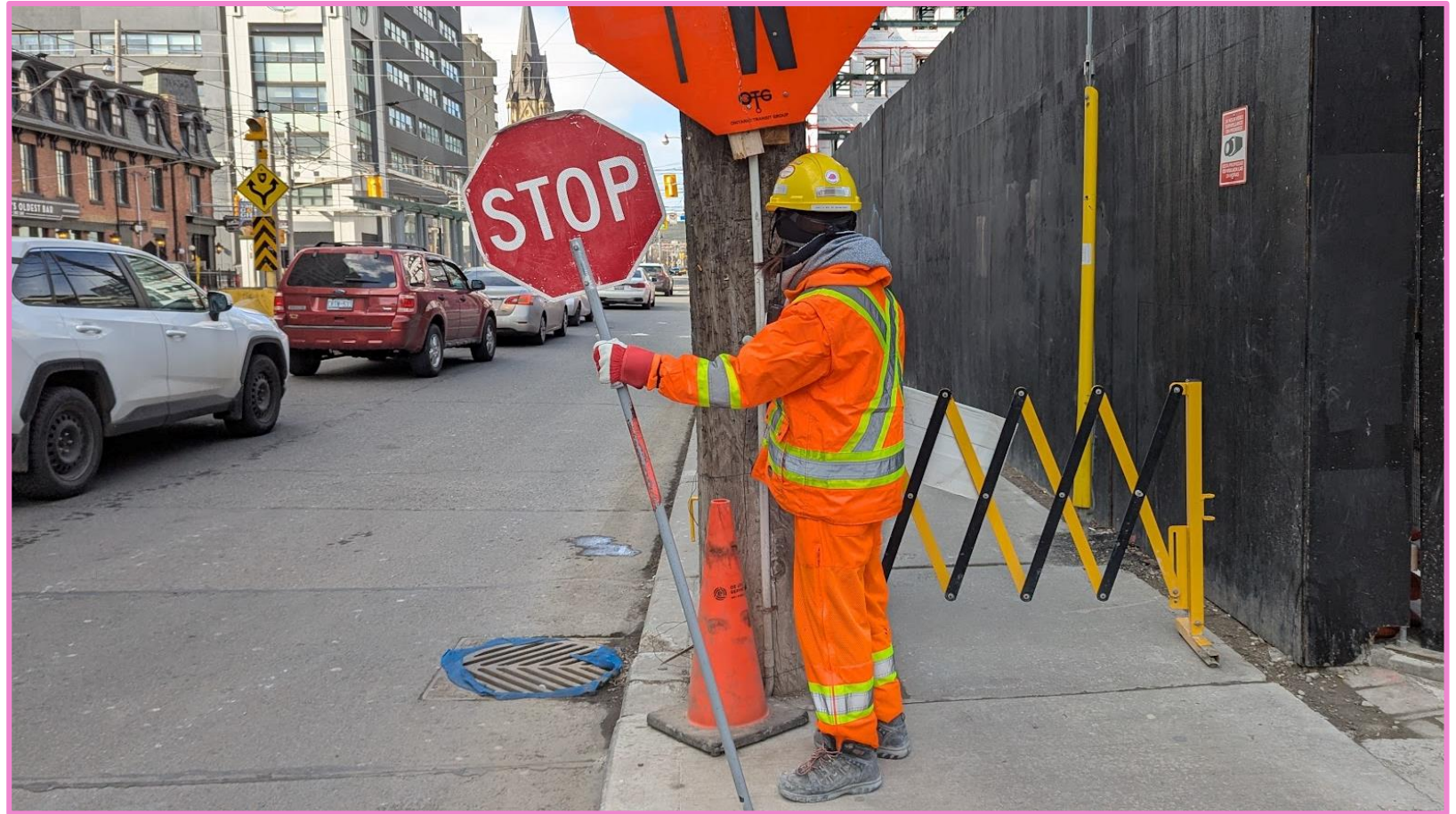
Construction vehicles and traffic being controlled by traffic flag persons, ensuring safe exit and entry into the King-Bathurst site.
