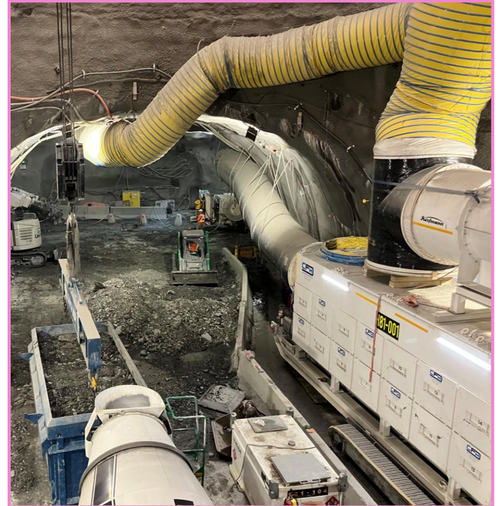
“Duduster” machine keeping the air clean in the station cavern at King-Bathurst
