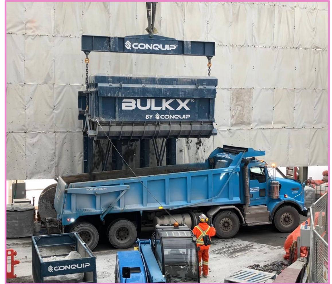
A self-dumping bin loading up a dump truck with excavated materials at King-Bathurst site.
