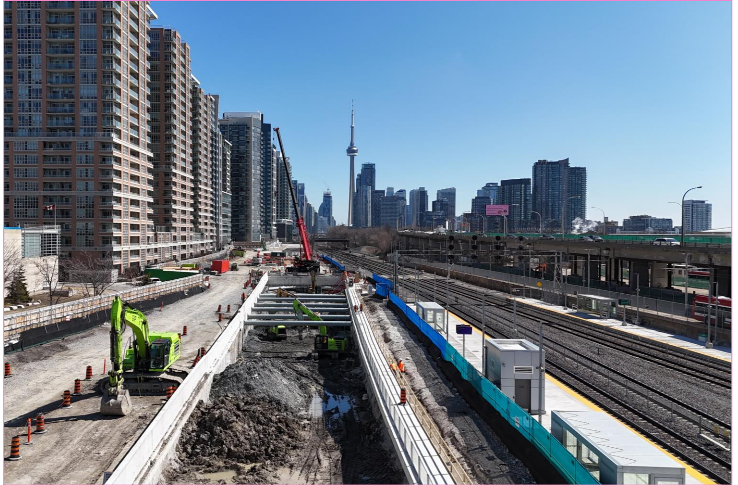
Ontario Line portal walls and struts, ensuring structural integrity as crews excavate.
