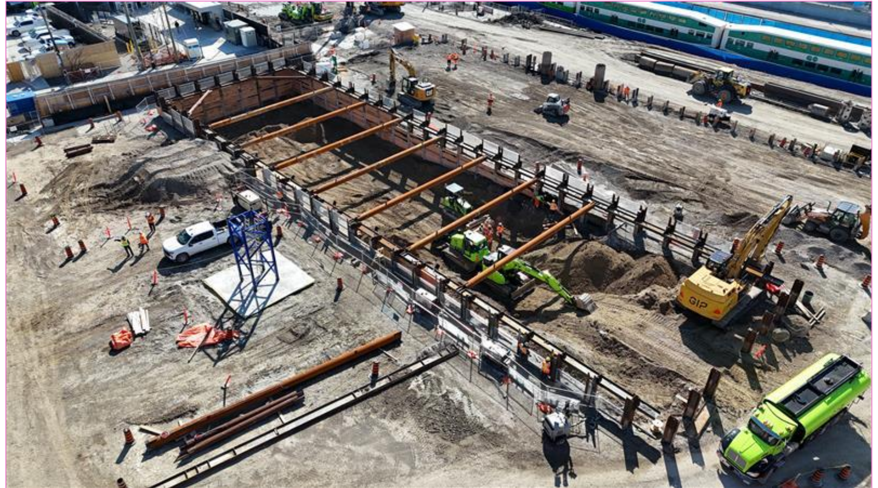
Support piles being installed to support the future north main entrance building.
