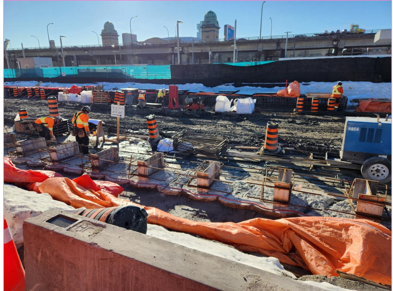
Capping beam work at the portal excavation area, ensuring horizontal stability to the top of below ground support beams.
