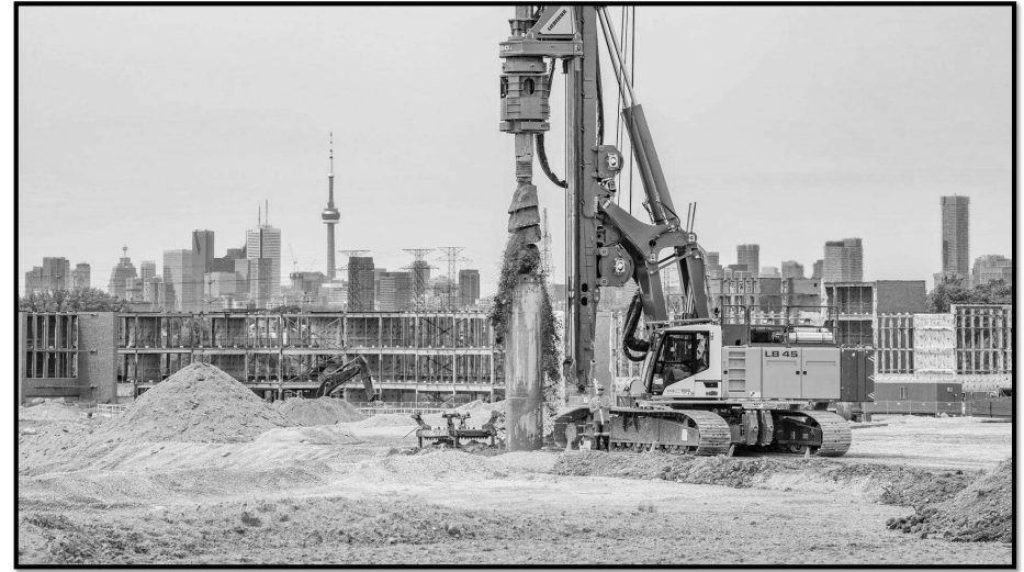
Example of caisson foundation Source: Liebherr Group
