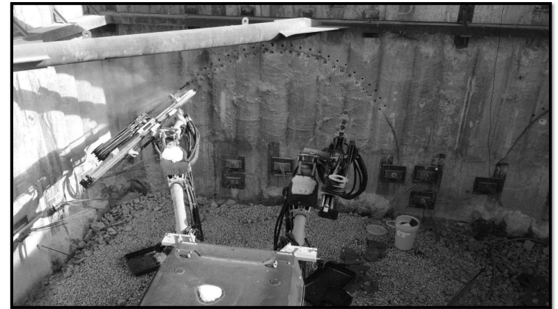
Close-up view of pipe umbrella installation in progress, showing drilling equipment and marked arc pattern on a concrete wall where steel pipes are being installed.
