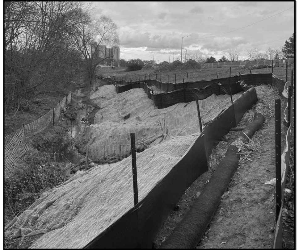
Double silt fencing at the elevated guideway construction site
