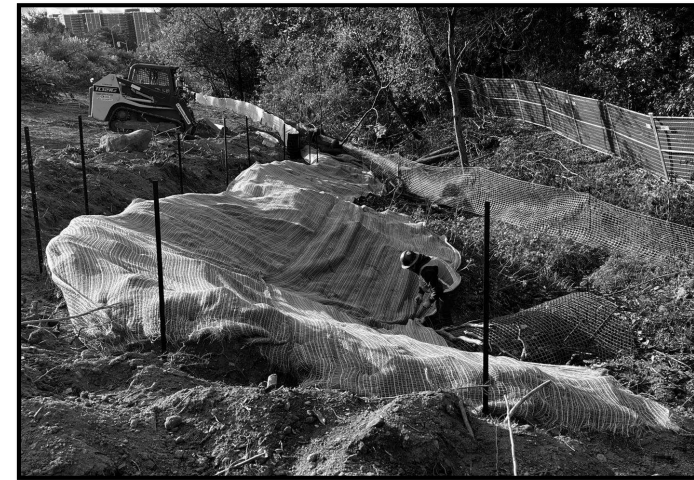
Erosion control blankets being installed at the elevated guideway construction site
