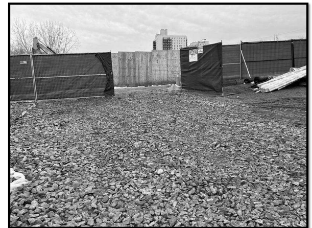
Mud mats at the elevated guideway construction site
