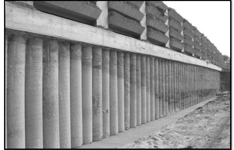
Example of secant pile wall Source: www.geotech.hr
