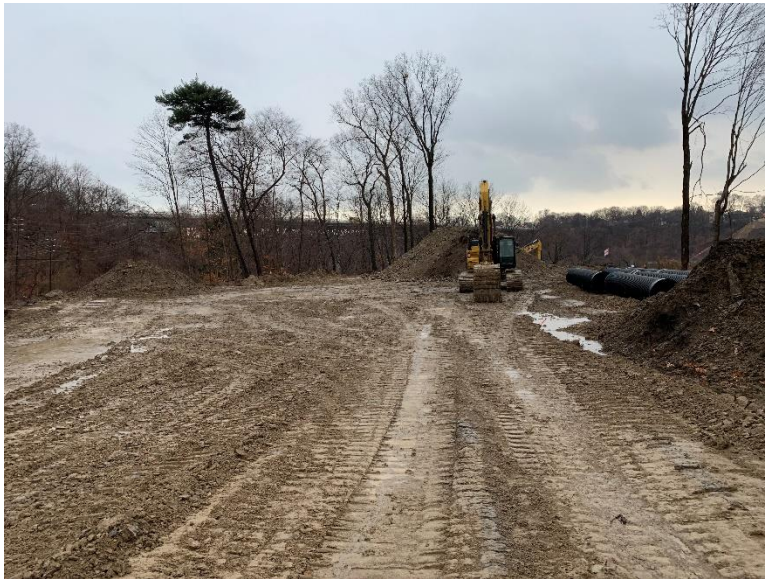
Figure D-7: Construction Compaction (left) Surface rooting often evidence of soil compaction (right)
