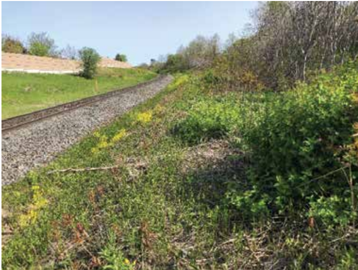
Figure 6-1: Photos Illustrating Clear Sightlines and Vegetation Management Zones within Non-Electrified Corridors as Required for Rail Safety and Daily Operations
