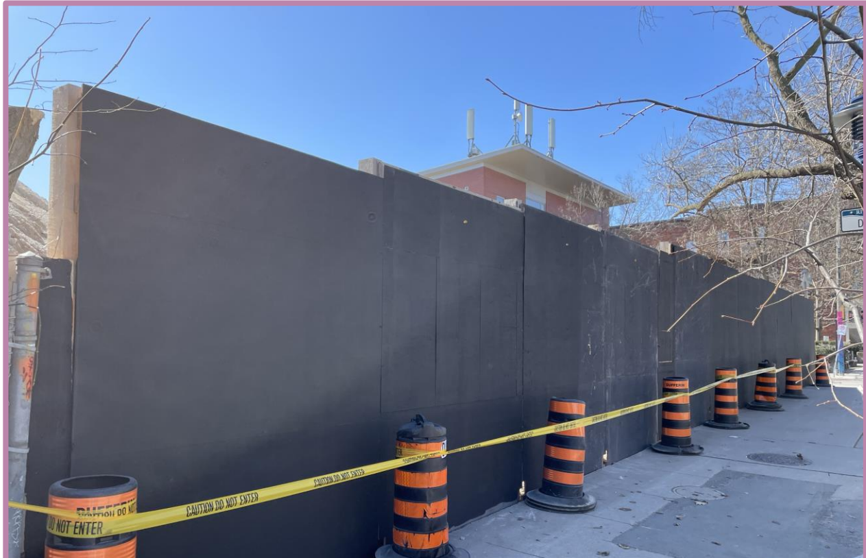
Noise barrier installed along Queen Street East
