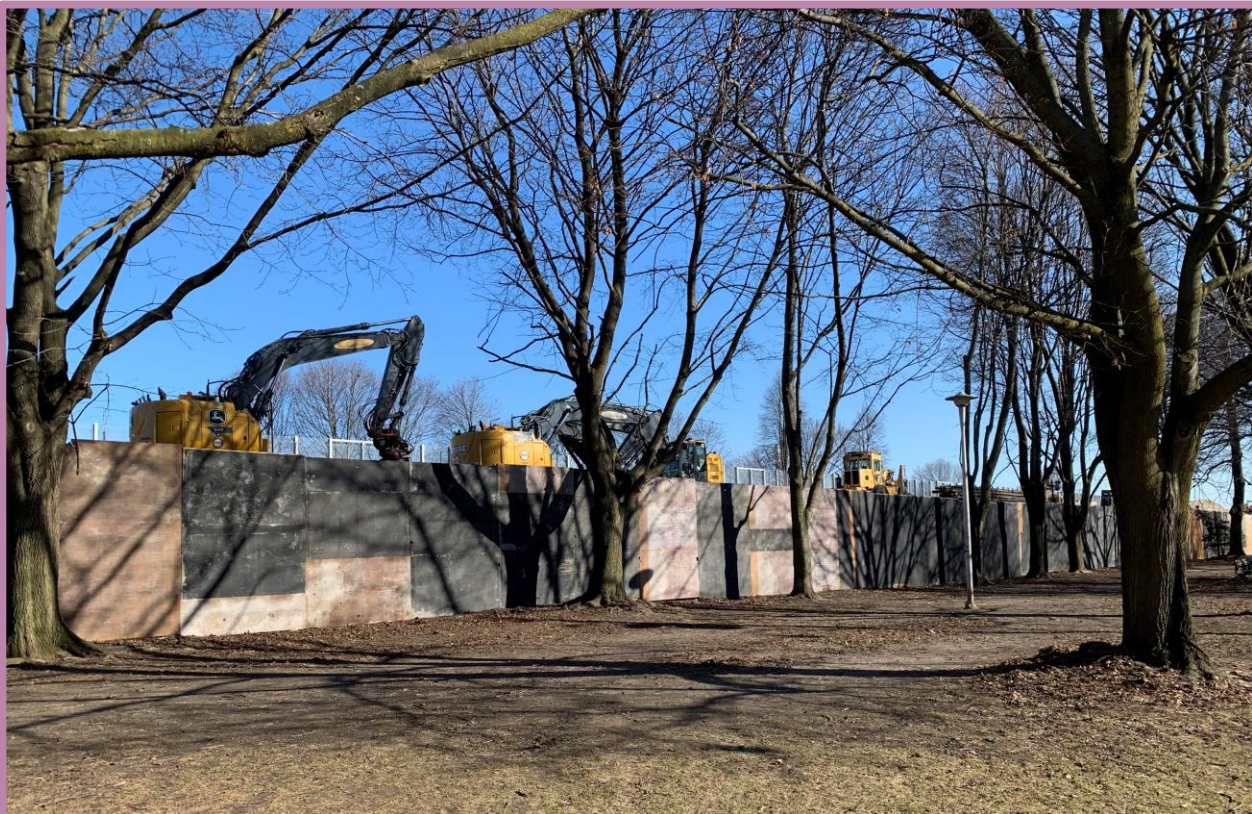
Solid noise barrier installed at Wardell Street (approx. 150m)
