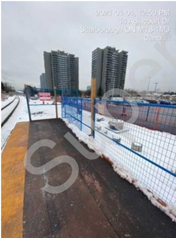
Photo 10: Temporary mini platform with non-slip coating
