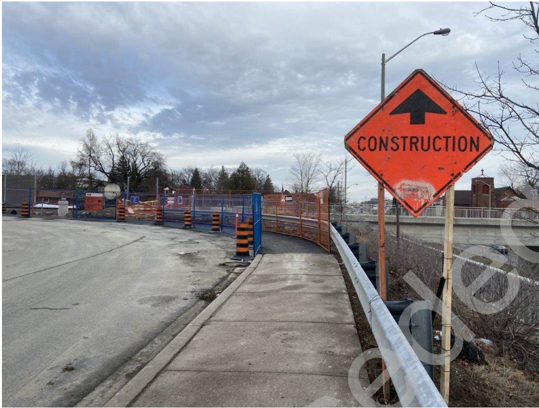
Photo 5: Temporary walkway delineated from roadway with fencing
