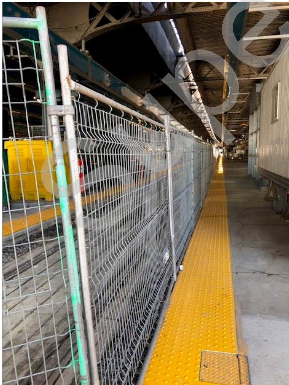
Photo 8: Fencing designed to maximize space on open platform
