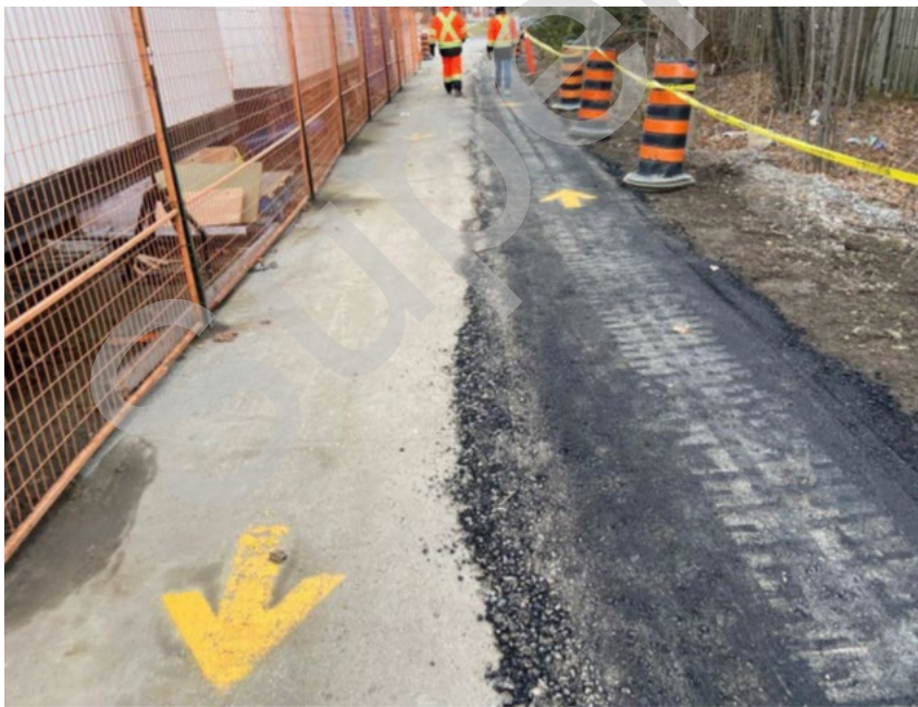
Photo 6: Temporary walkway widened to 1800mm
