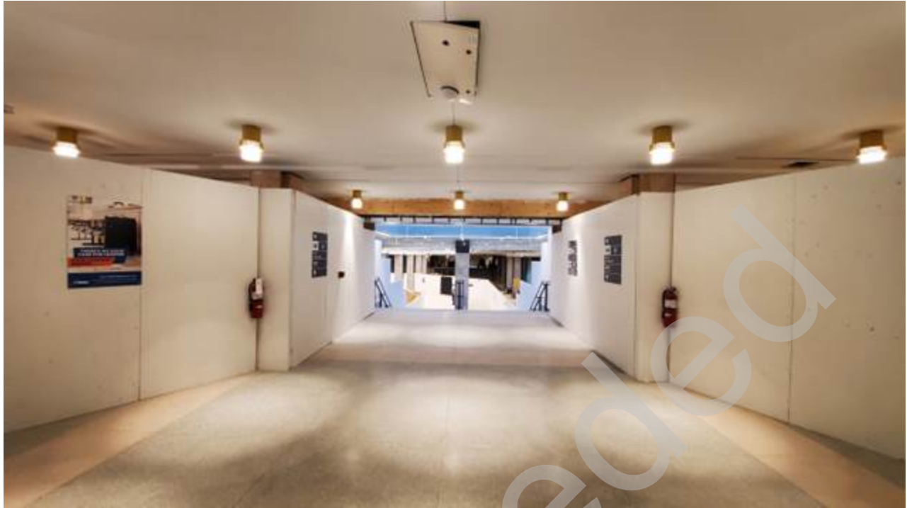
Photo 2: Hoarding is painted, has a smooth profile, and uses full sheets. Damaged sheets are replaced.
