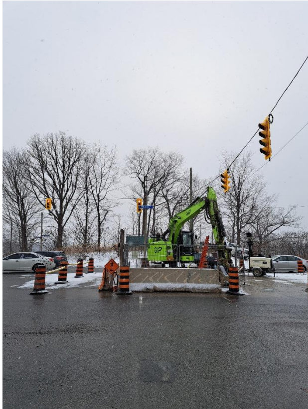
Watermain Valve Installation at Millwood & Overlea in January.
