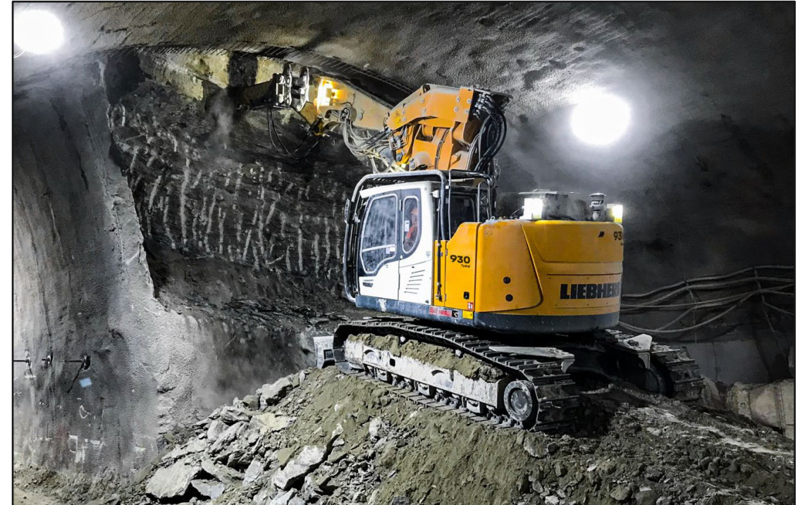
Example of tunnel excavator that will be used at the sites at Corktown. Picture is for reference only.
