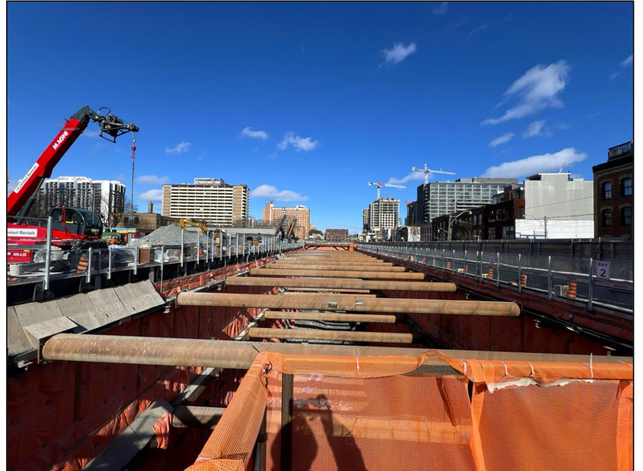
View of the struts and walers system looking east
