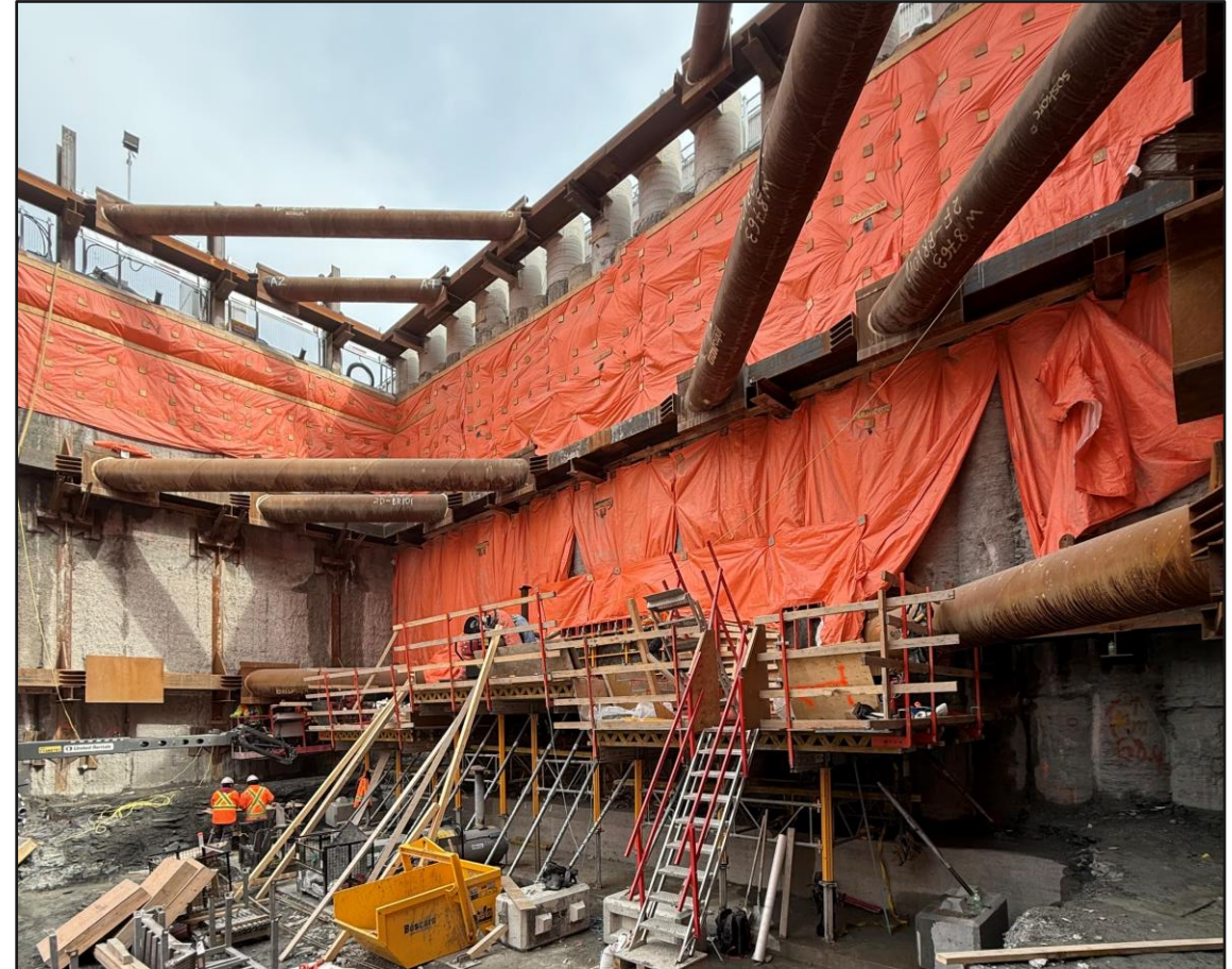
Forming the arch beam for concrete works in the north shaft
