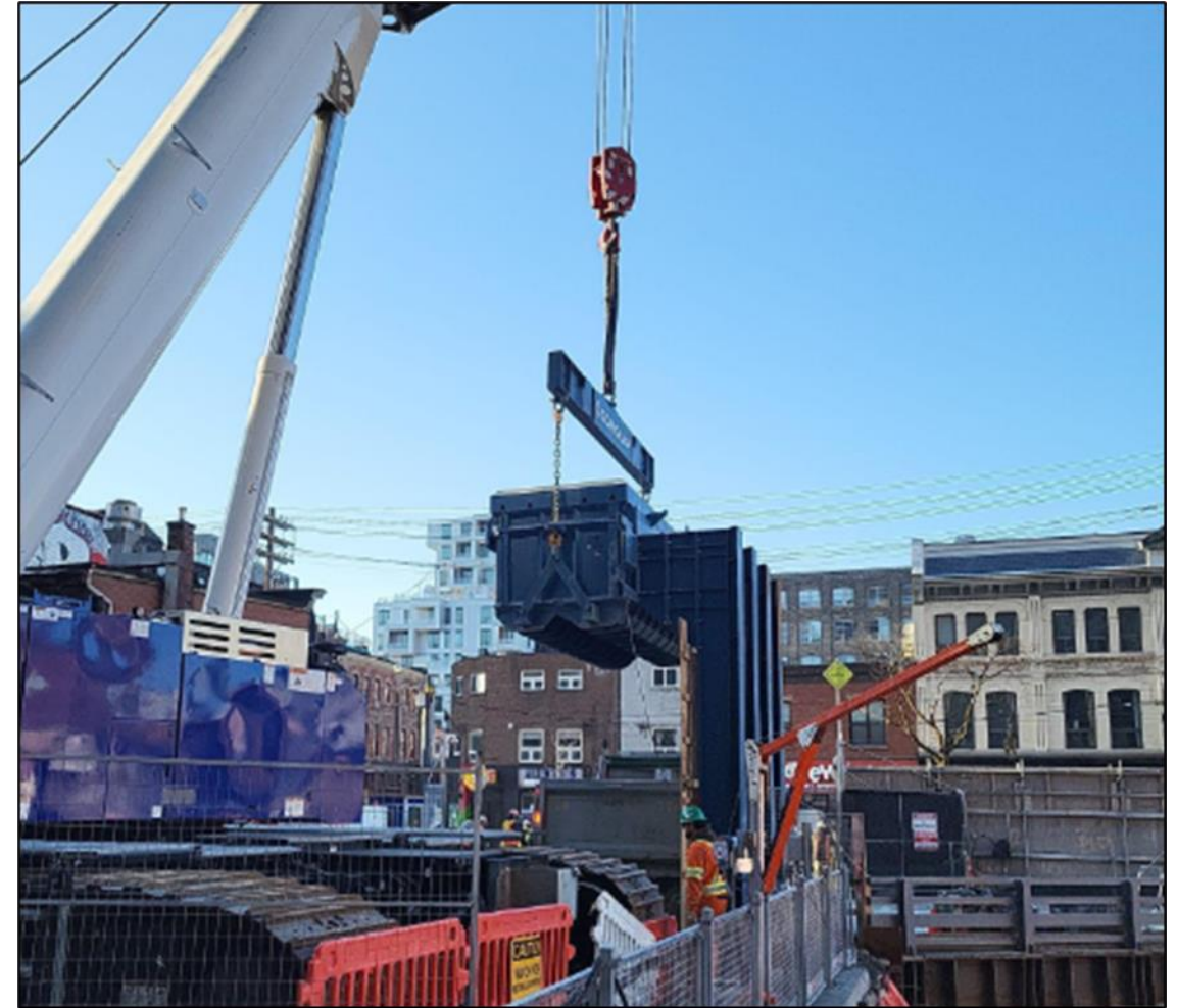
A self-dumping bin loading up a dump truck at Queen-Spadina south site with excavated materials.
