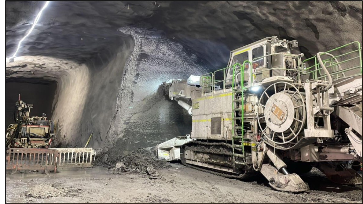
Roadheader machine removing rock to create the cavern at the future Queen-Spadina station site.
