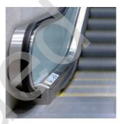
Figure 4-33: Precedent image demonstrating stainless steel enclosure and frosted glass balustrade adjacent to wall.
