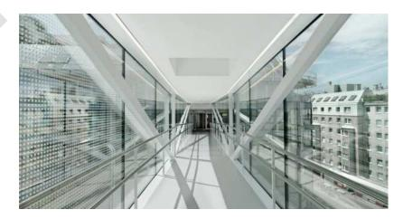
Figure 4-52: Precedent image demonstrating a pedestrian bridge using ceramic frit as a shading strategy. Bridge in Vienna, Austria, by SOLID architecture. Image Courtesy Günter Kresser
