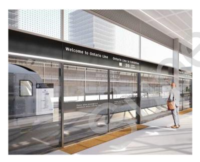
Figure 7-6: View from the elevated platform typology demonstrating the relationship between the platform edge doors, digital signage and lighting. Renders are representational only.
