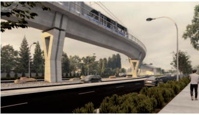
Figures 4-53 to 4-54: Precedent images demonstrating minimizing the impact of an elevated guideway in the public realm through tapering of elements, continuity of horizontal lines, concealing of clutter, an maximizing slope of guideway at portals to demonstrably minimize obstructions at grade. Valley Line LRT, Edmonton, Alberta, by Dialog.
