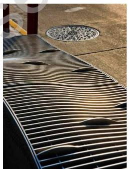
Figure 3-62: Tunnel Ventilation Shafts with Integrated Seating
