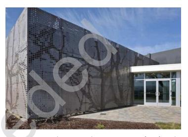
Figure 4-25: Precedent image demonstrating use of perforated metal cladding with creative perforation patterns on an EEB in the public realm. One Workplace, Santa Clara, California, by Design Blitz. Image Courtesy © Bruce Damonte
