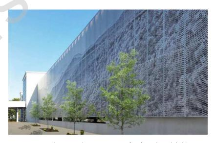
Figure 4-16: Precedent image demonstrating use of perforated metal cladding as an exterior feature element, creating a site specific station identity through printing of imagery. Ashville Regional Airport, Fletcher, North Carolina by Gresham Smith and Partners
