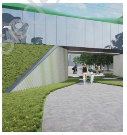
Figure 3-57: Retaining Wall - Coloured and pattern concrete
