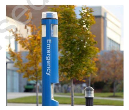
Figure 3-64: Exterior Emergency Blue Light Station
